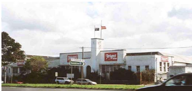
Image 8. Former Southern Can Company, Dimmeys/Forges, 240 Geelong Rd, Footscray West Source: HLCD Photo Sept 2004
