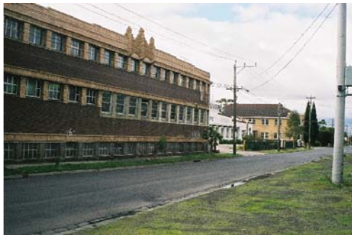
Photo 3. View of site from Cross Street looking east
