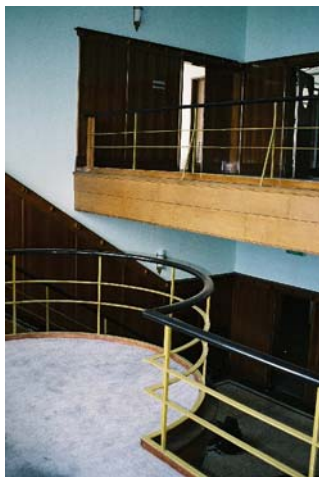
Photo 15 The two stair landings in the foyer of the 1939 Administration Building
