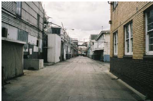
Photo 10. View down main roadway from the entrance
