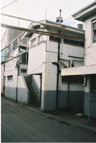
Photo 21 Engineering offices, part of the Staff Amenities Building
