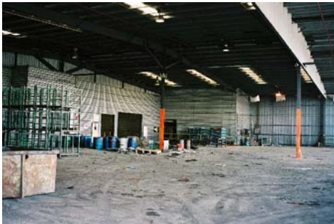
Photo 23 Steel portal frame storage area (labelled 10 on site plan)
