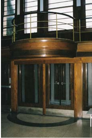
Photo 17 Revolving door and landing in foyer of 1939 Administration Building
