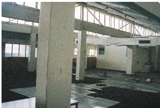
Photo 8. Main office space in 1934 Office Building
