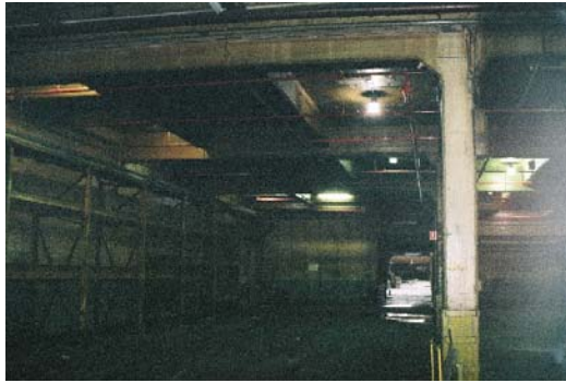
Photo 13 Interior view cinder block storage section (Area 3b on site plan)
