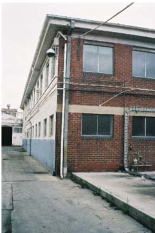
Photo 20 Staff Amenities Building
