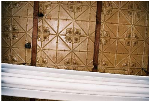
Photo 6. Pressed metal ceiling in showroom
