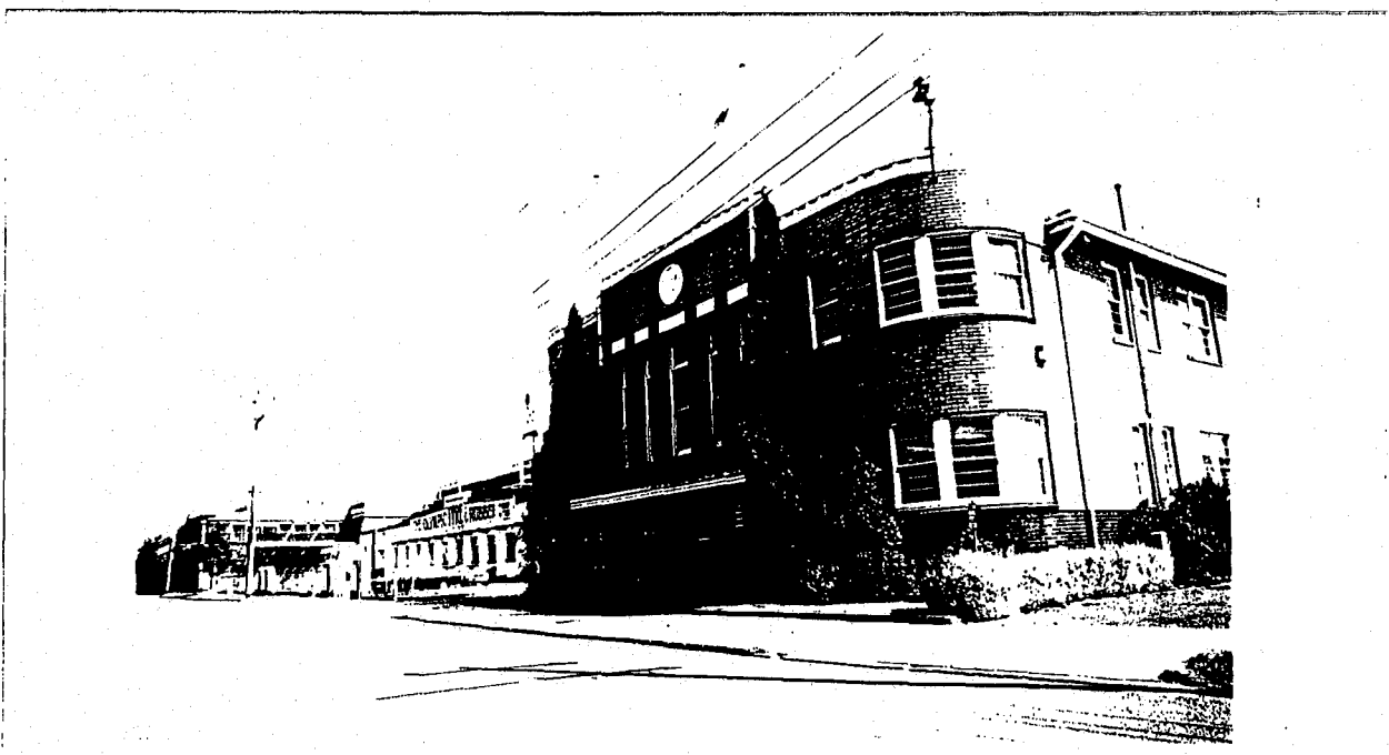
4 - 32 56-84 Cross Street, foundation stone laid 1939
