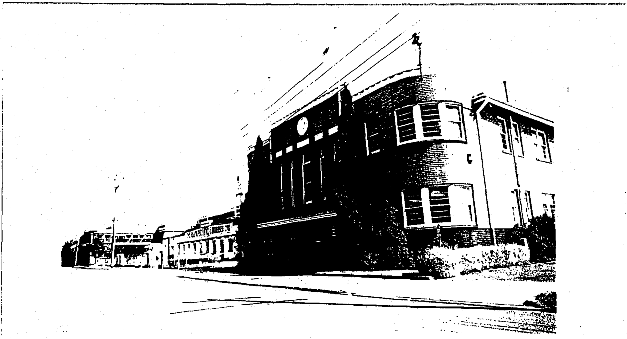
4 - 32 56-84 Cross Street, foundation stone laid 1939
