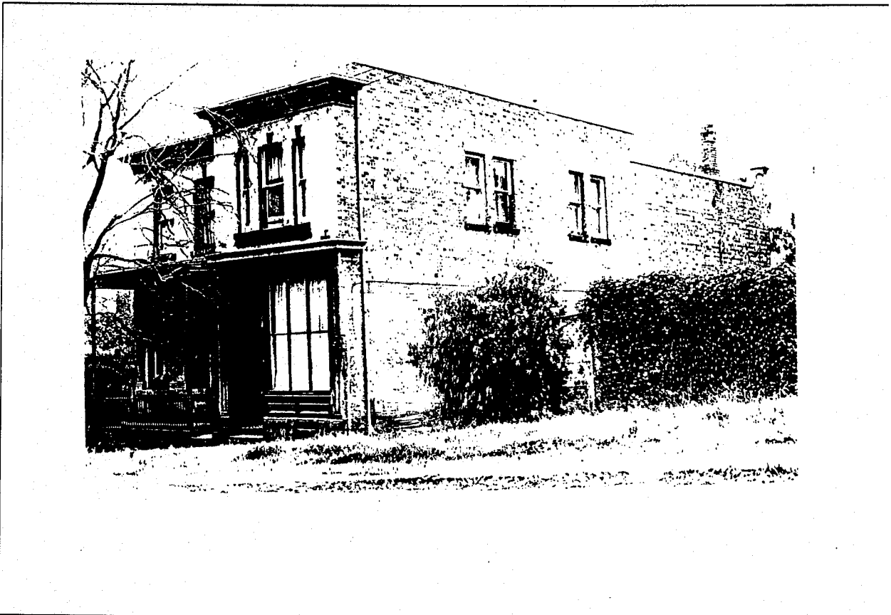
4-78 98-100 Moreland Street, shop and residence at front, store and bakery at rear facing a carriage yard.
