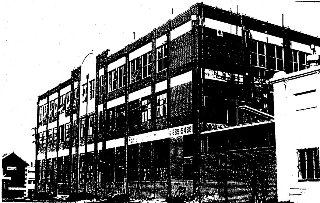
4-77 91 Moreland Street, 3-storey c1934-5 wing, shows steel window and rectilinear forms of the 1930s but with the added Edwardian character of the raised parapet entablature
