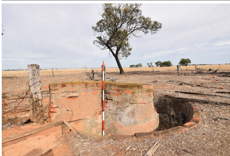
Plate 2: Sheep dip showing coursed bricks and render - view northwest
