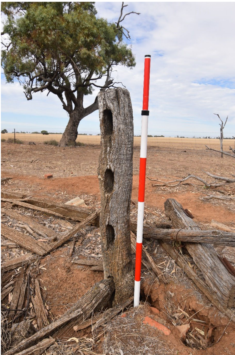
Plate 5: Example of hand cut timber post with remnant in-situ timber rail - view southeast
