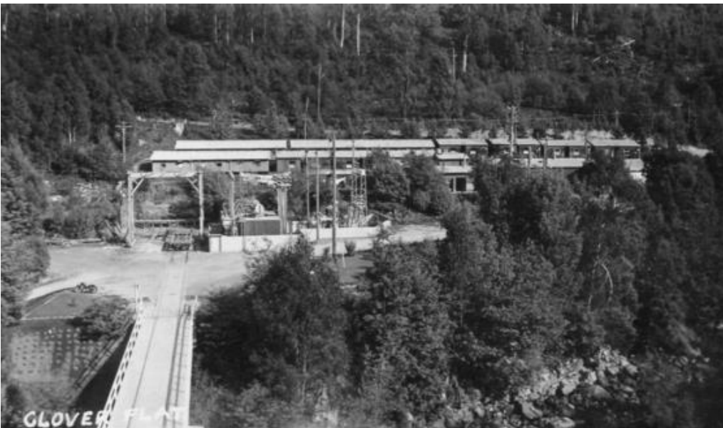
Figure 12 Workers' camp location with the electrical infrastructure installed (Photographs - SECV - Clover Power Station, 1940s)
