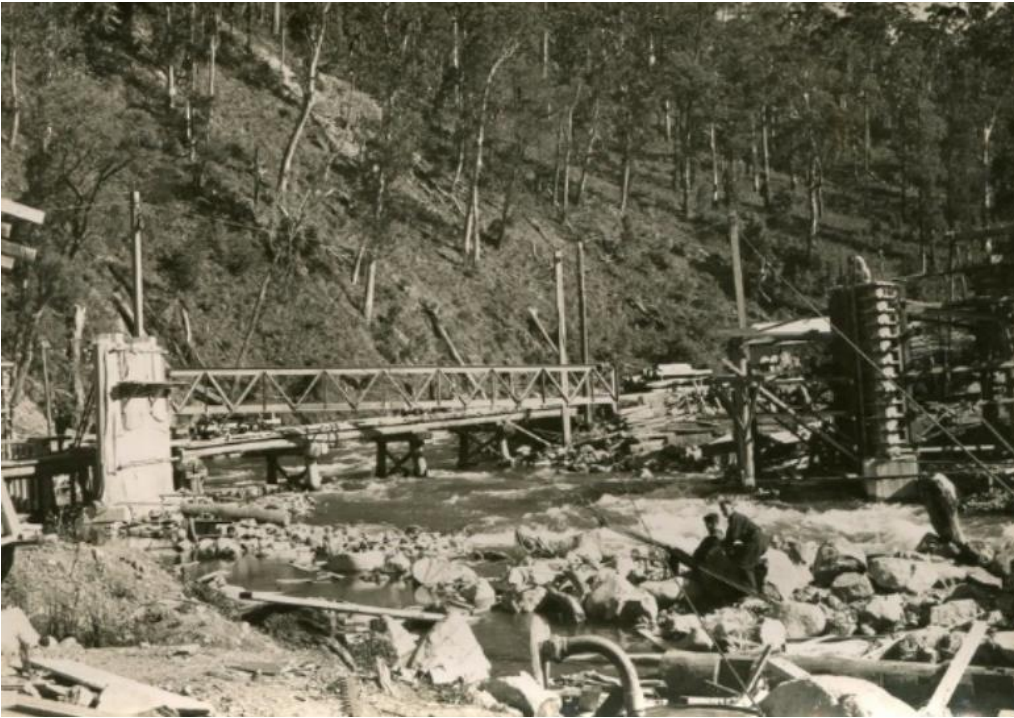
Figure 7 Construction of Clover Dam Power Station bridge, with the power station site to the right of the photograph and the piles for the bridge under construction (Photographs - SECV - Clover Power Station, 1940s)
