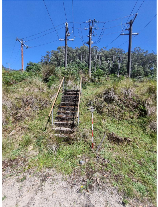
Photograph 12 Existing concrete steps leading down from the lower benched area to the level of the power station (facing west, D.Carpenter, 14 February 2024).
