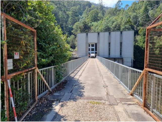
Photograph 14 Clover Power Station, picture provided for context and reference purposes (facing east, D.Carpenter, 14 February 2024).
