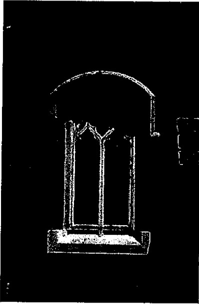
Photo 3.44a: Exterior, east elevation. Detail of window 9.
