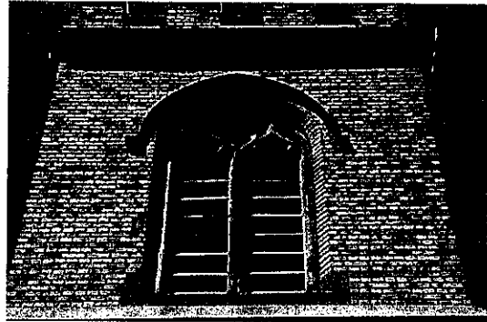
Photo 3.52: Exterior, north elevation. Detail of tower ventilation opening.
