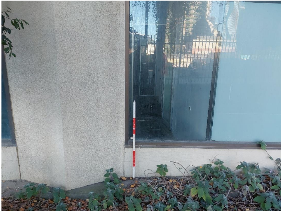
Figure 7: Demonstrating exterior ground surface, towards centre of building, is significantly higher than interior (see Figure 5), view north
