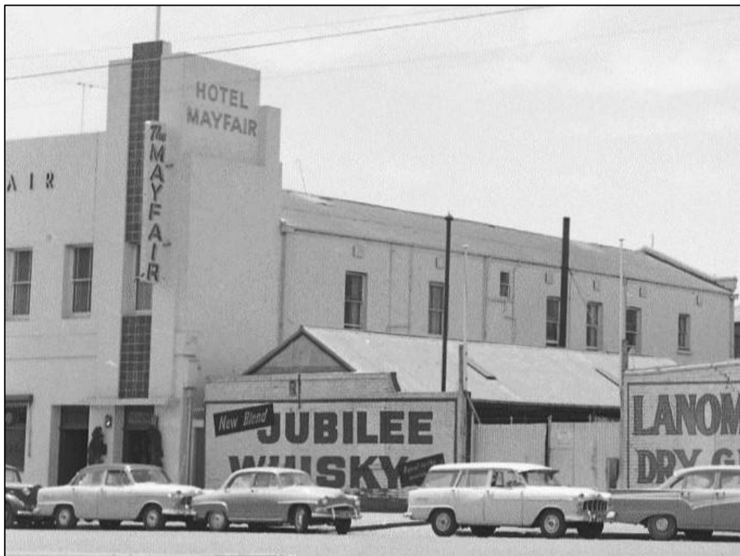
Figure 14: The Hotel Mayfair (former Harvest Home Hotel), as depicted in a 1956-65 photograph, view north-east. Source: City of Melbourne Collections
