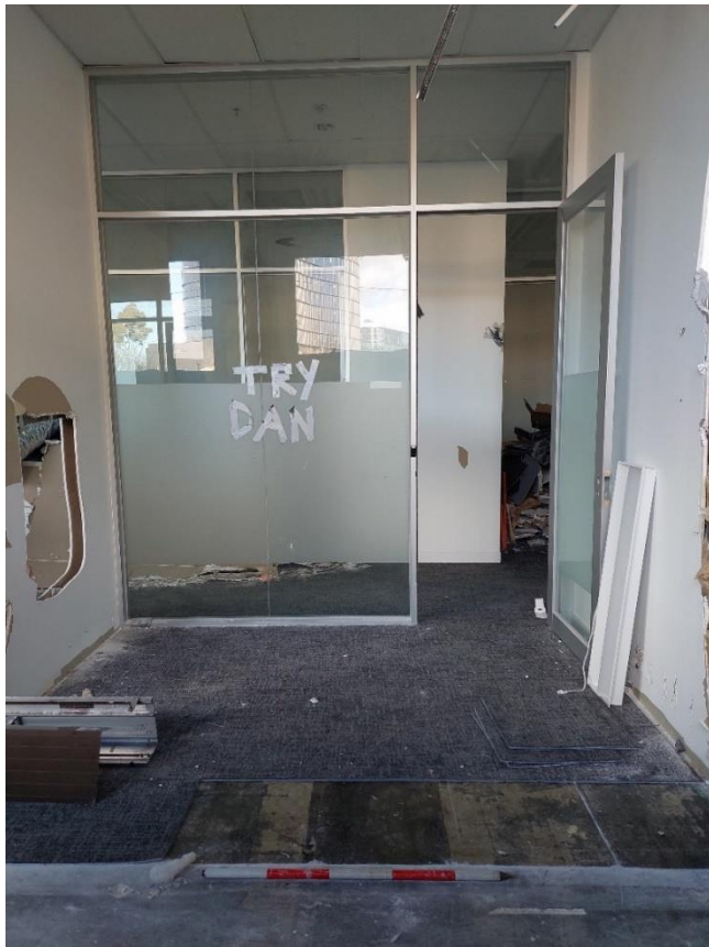
Figure 5: Interior rooms of 766 Elizabeth Street, view north
