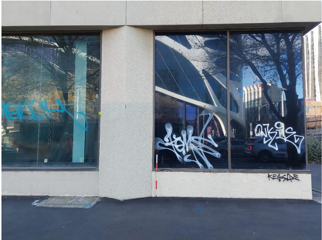
Figure 2: Exterior of extant office building fronting Elizabeth Street, view east
