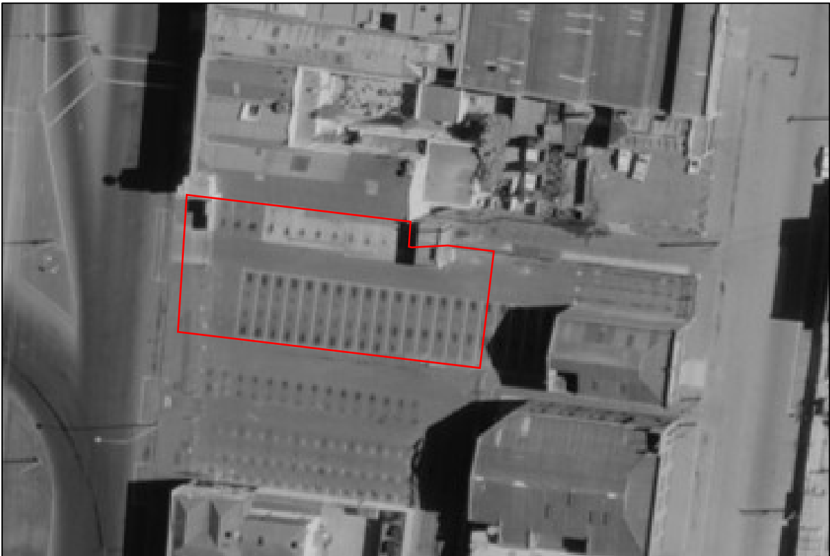
Figure 20: The Former Sachs Brothers' Coach Factory (in red) in a 1969 aerial photograph (Source: Landata)
