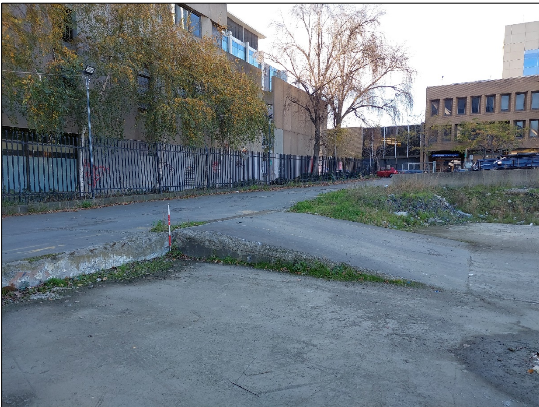
Figure 5: Modern vehicle access ramp between the naturally sloping access road (background) and the 1980s cut (foreground), view east (A.Valka, 26/06/2024)
