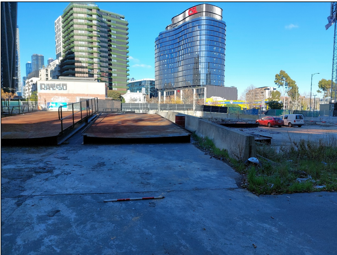
Figure 7: The eastern end of the Former Sachs Brothers' Coach Factory, view south-west, showing the section of the site located above the 1980s cut (A. Valka, 26/06/2024)
