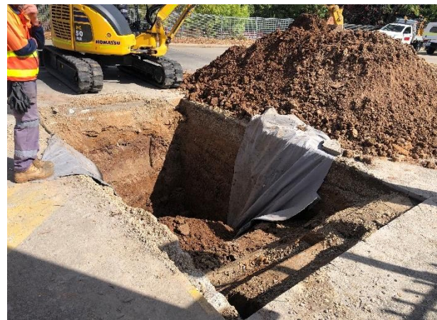
Plate 4.6 Covering wooden beam and bricks with geofabric before reburial
