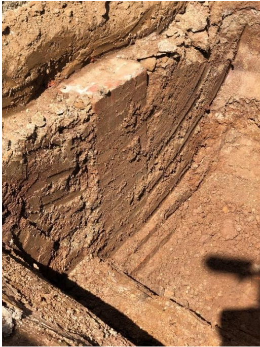
Plate 4.3 Redbrick foundations with intact step down brick formation, 2 m below carpark surface
