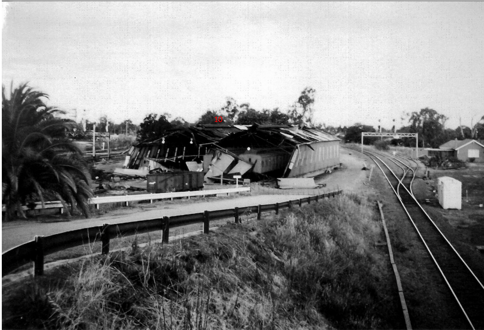
Plate A.16 Locomotive workshop in 1994 following collapse during storm
