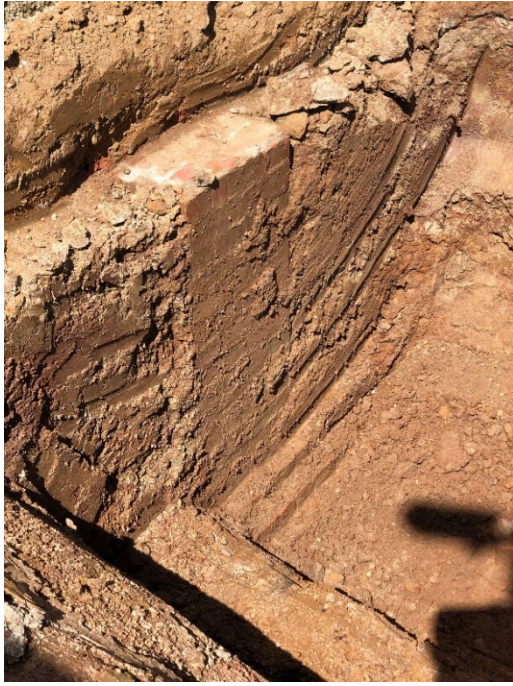
Plate 4.5 Redbrick foundations with intact step down brick formation, 2 m below carpark surface
