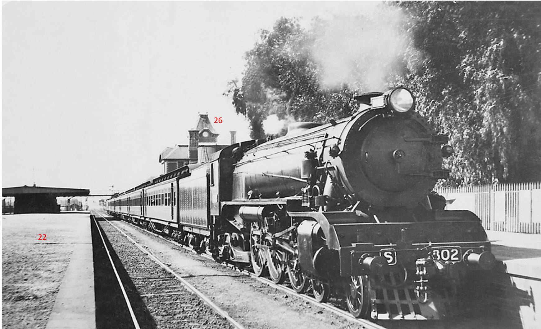
Plate A.17 Benalla Station showing the second platform on the left, pre-1935.
