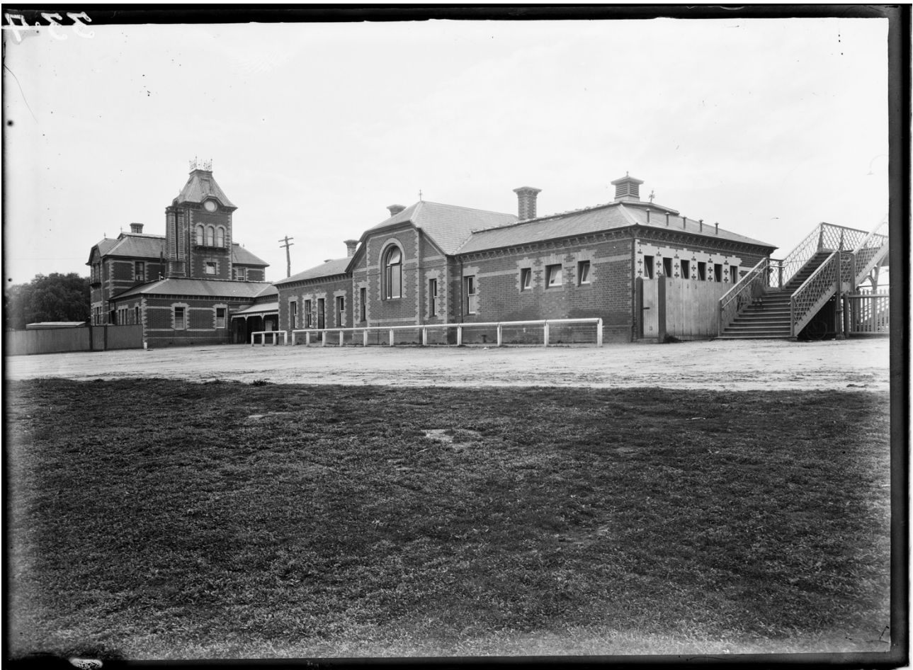
Plate 2.2 Undated early 20th century photo of Benalla Station showing the refreshment room extension, footbridge and a possible vehicle protection barrier in front of the station
