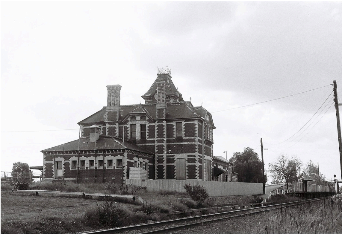
Plate 2.6 1960s view of new rail line between station and Mackeller Street
