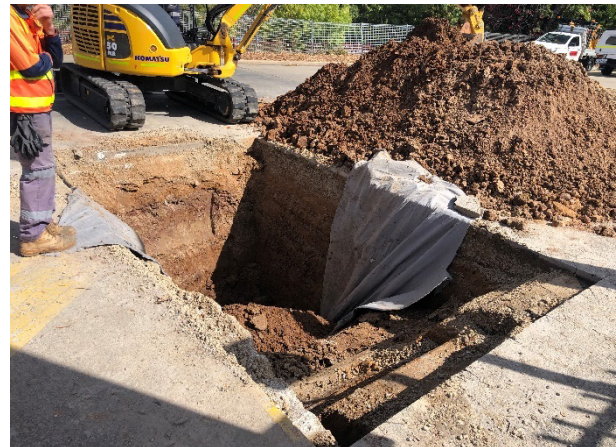
Plate 4.8 Covering wooden beam and bricks with geofabric before reburial
