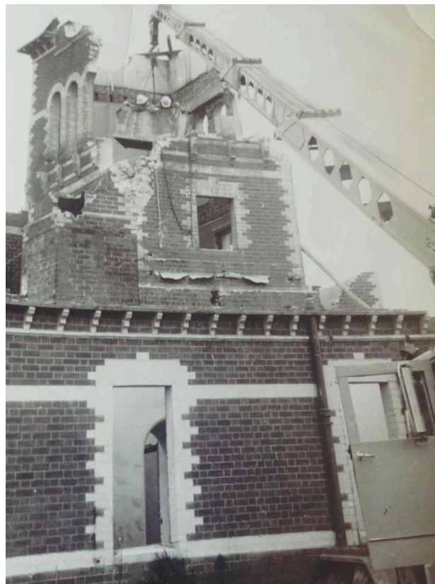
Plate 2.9 Demolition of the clock tower at Benalla Railway Station, November 1974
