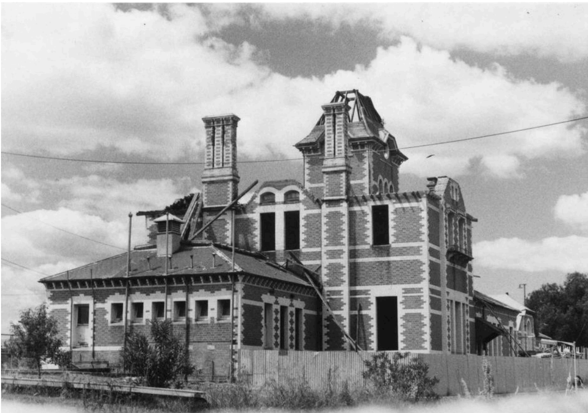
Plate 2.8 Demolition of the Refreshment Rooms 14 November 1974
