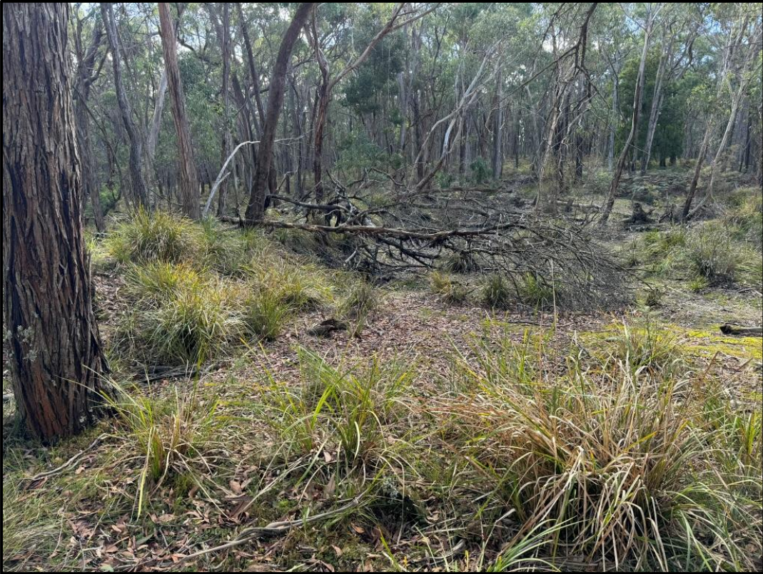
Embankment of the smaller dam
