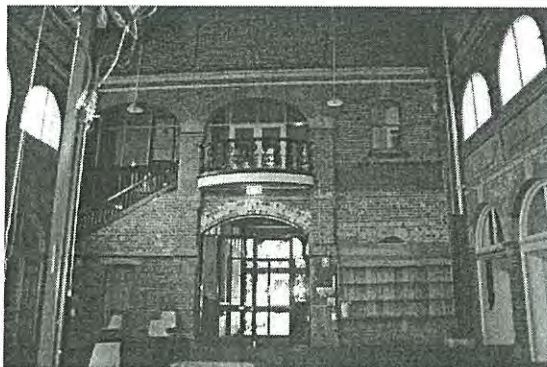
Photo 3.67: Interior, Exchange Hall (space H01). View of west wall. Note the altered central arch with introduced aluminium framed and glazed partition with double doors.
