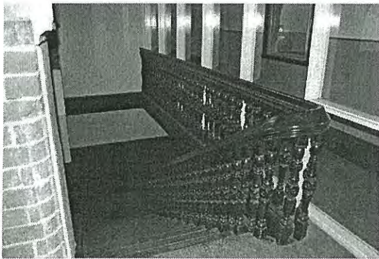
Photo 3.39: Interior, Landing & Stairs (space FF12). View of original upper flight of stairs. Also note the introduced timber and glazed partition wall to the west (right of stairs).
