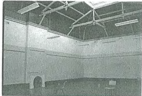
Photo 3.84: Interior, Call Room (space CR01). View looking north-east showing large timber lined ceiling with Queen Post trusses and lantern light, and the central fireplace on the north wall.
