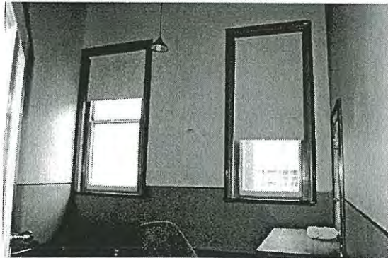
Photo 3.55: Interior, Office (space FF07), showing west wall and original timber framed double hung windows.
