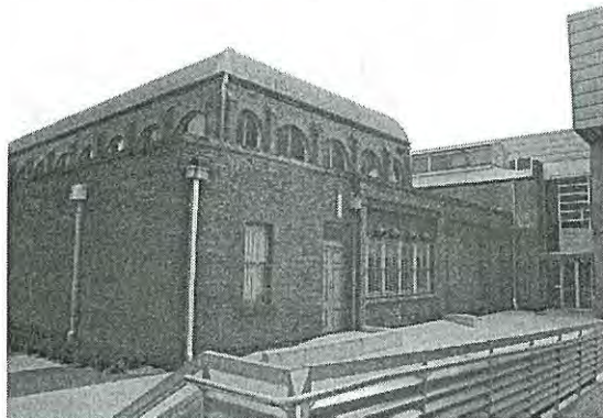
Photo 3.11: Exterior, Exchange Hall, east elevation (and part south elevation).
