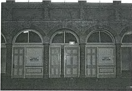
Photo 3.59: Interior, Exchange Hall (space H01). View of introduced panelled timber and glazed partitions on north wall, screening the ladies' and men's toilets. These partitions appear to be a reconstruction of the original design. The wider single six panelled timber door is original.
