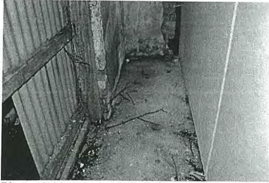
Photo 3.99: Interior, Men's Toilets (space T01). Detail of area of demolished toilet cubicle. Note the introduced raised concrete slab and the build up of debris within this open space.
