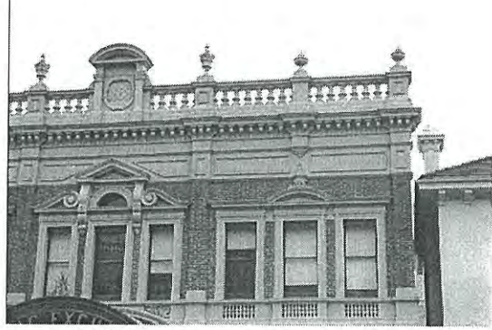
Photo 3.02: Exterior, Front Pavilion, detail of west first floor façade and parapet.
