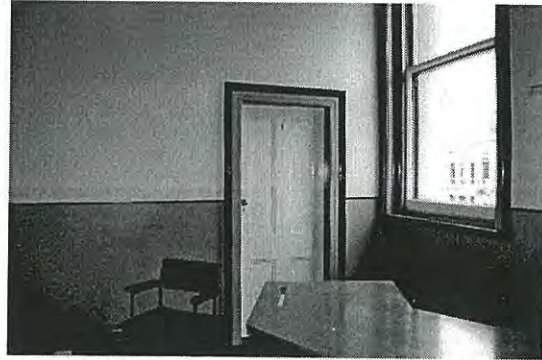
Photo 3.54: Interior, Office (space FF07). View looking south-west.
