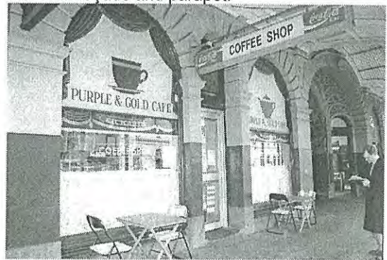
Photo 3.04: Exterior, Front Pavilion, detail of arcaded ground floor shopfronts on the west façade.
