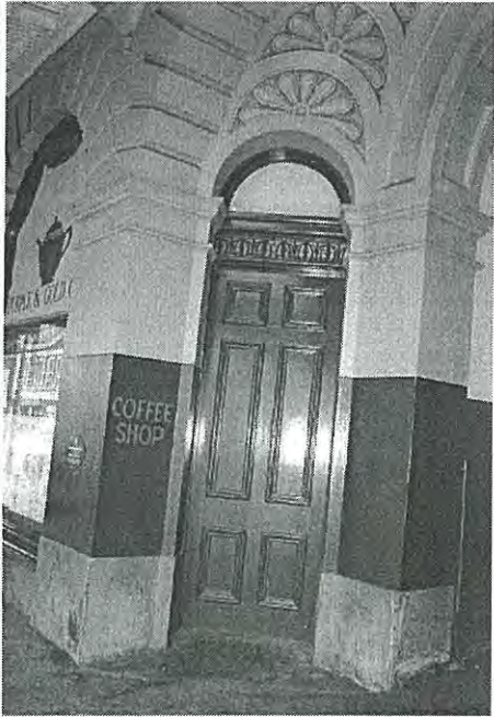
Photo 3.07: Exterior, Front Pavilion, detail of reconstructed six panelled timber door with round-arched fanlight above. This door is on the north side of the base to the springing of the entrance arch. Note the decorative floral motifs in the arch. Also note that the fanlight has been painted over to obscure introduced lowered ceiling within.
