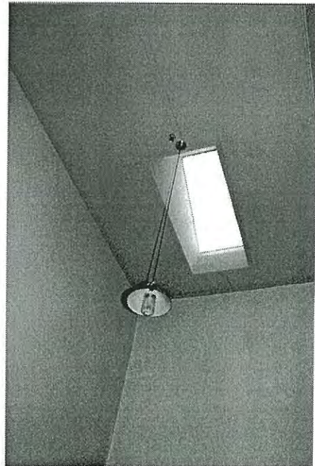
Photo 3.46: Interior, Office (spaces FF01-02). Detail of original (altered skylight), north end.
