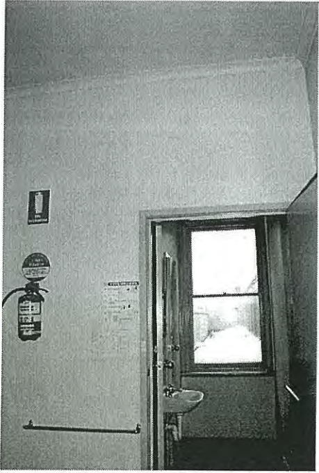
Photo 3.47: Interior, Kitchen & Toilets (space FF03). View looking east showing introduced cubicle walls in the foreground and original timber framed double hung window opening in the background.
