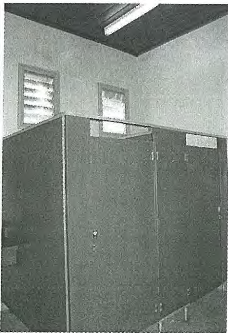
Photo 3.77: Interior, Ladies' Toilets (space B08a). Detail of introduced toilet cubicles and windows (in the background).
