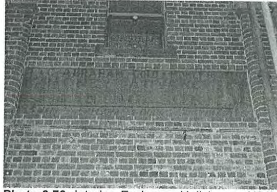
Photo 3.70: Interior, Exchange Hall (space H01). Detail of early signage below first floor window on west wall (north end).
