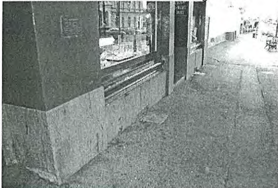
Photo 3.09: Exterior, Front Pavilion, detail of raised ground level outside shopfronts.
