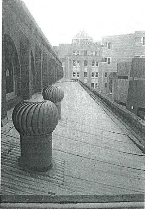
Photo 3.17: Exterior, Exchange Hall, south elevation (clerestorey level), west end, showing galvanised ventilation stacks.
