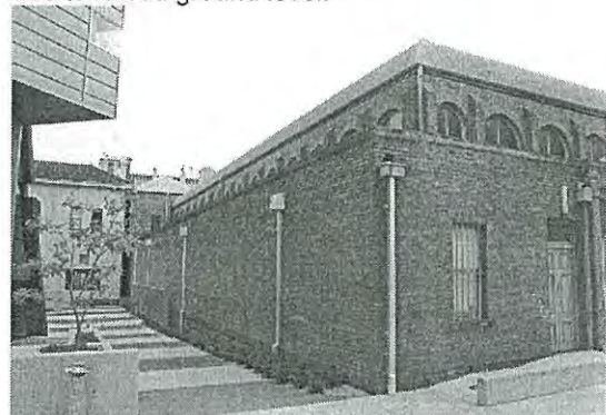
Photo 3.12: Exterior, Exchange Hall, south elevation (and part east elevation).
