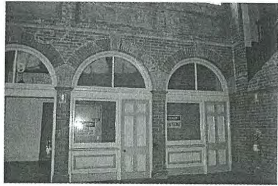
Photo 3.66: Interior, Exchange Hall (space H01). Detail of western-most booth arcades on south wall. These booths have been converted into an electrical substation. The panelled timber and glazed partitions appear to be a reconstruction of the original design.
