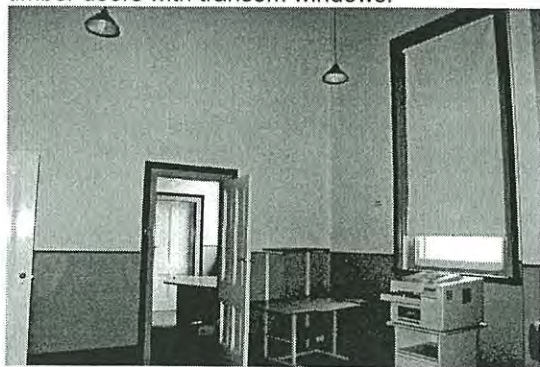
Photo 3.52: Interior, Office (spaces FF04-05). View looking south-west.
