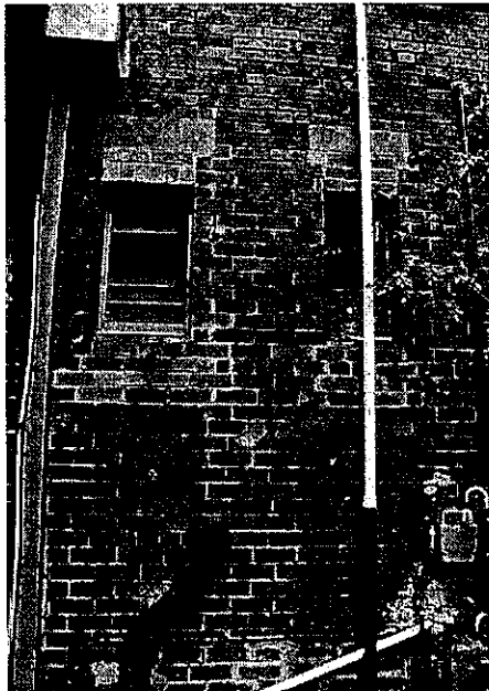
Photo 3.21: Exterior, Exchange Hall, part lower north elevation showing introduced toilet windows of ladies' toilets.
