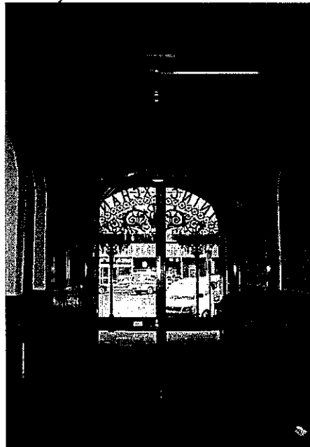
Photo 3.34: Interior, Entrance/Stair Hall (space FG05). View of west end showing introduced aluminium framed and glazed partition with double doors.
