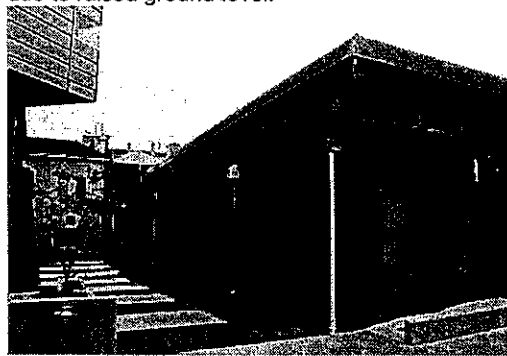
Photo 3.12: Exterior, Exchange Hall, south elevation (and part east elevation).
