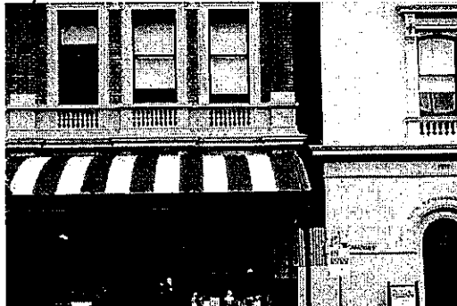
Photo 3.03: Exterior, Front Pavilion, detail of reconstructed verandah on the west façade.
