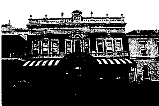
Photo 3.01: Exterior, Front Pavilion, West Façade.
