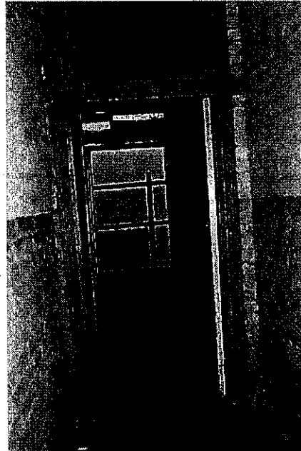
Photo 3.94: Interior, Passage (space T03). View looking north to Men's Toilet (space T01). Note the original timber framed doorway with transom window above, and the moulded timber architraves. Also note the concrete floor and evidence of dampness.
