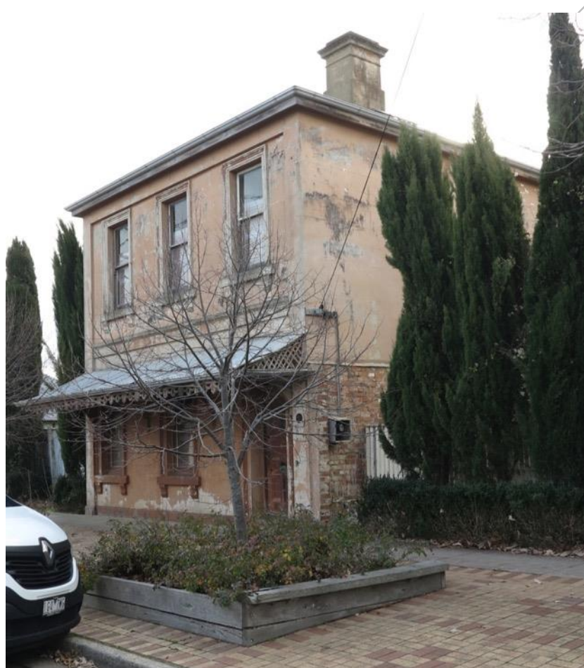
Facade of 140 Inglis Street, Ballan, July 2018. Photo by heritageALLIANCE
