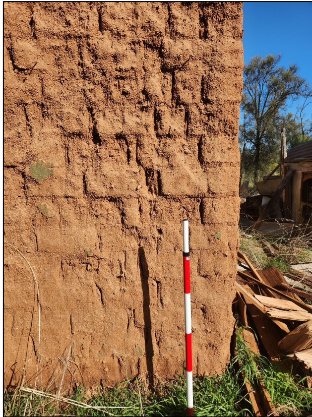
Figure 4: Detail of the mud brick wall construction of the Kerang-Quambatook Road Ruin, with patches of the outer paint coating visible (C. Lovell, 11/07/2023)
