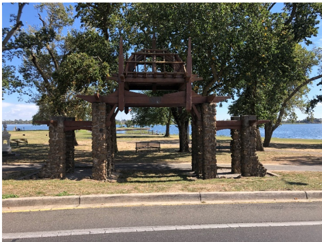
2022, George Tonner memorial pergola, constructed in 1925.
