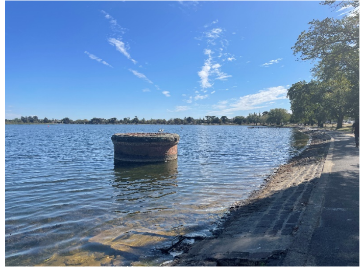
2022, Brick overflow well.
