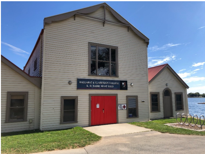
2022, Ballarat & Clarendon College boat shed (KD Baird Clarendon College Boatshed) (1896, restored c.1994).
