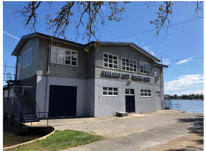
2022, Ballarat City Rowing Club boat shed (rebuilt 1950).
