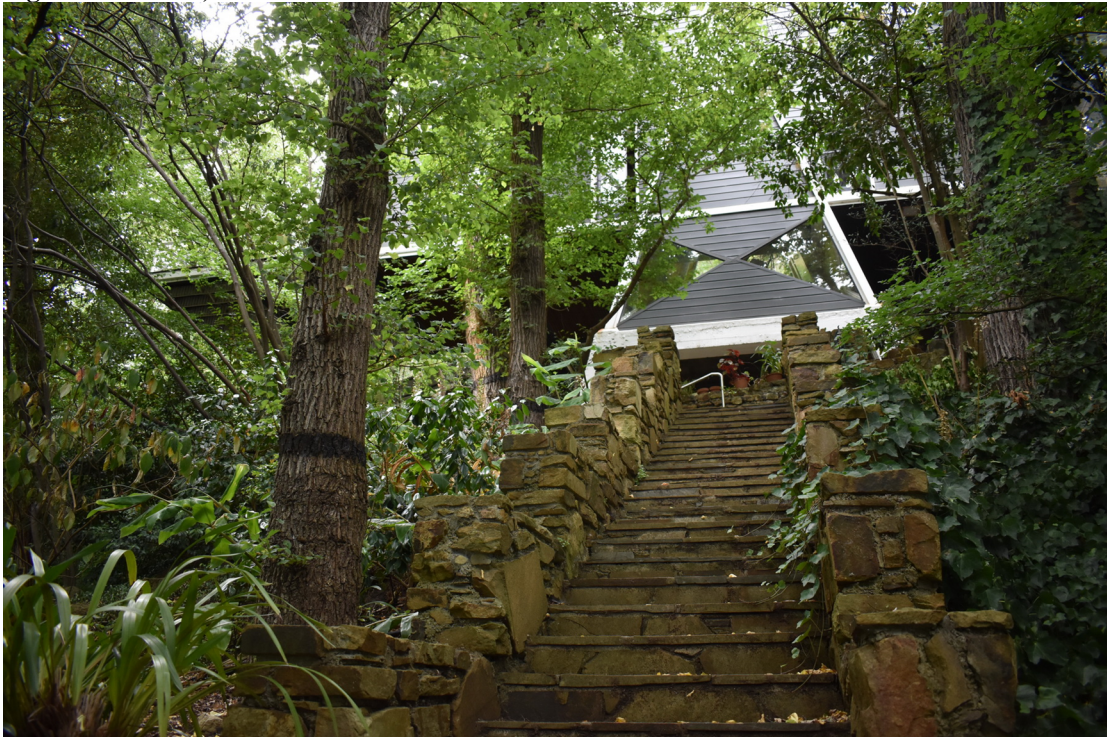
Figure 7. View of approach to River House from jetty, showing stone stairs.
