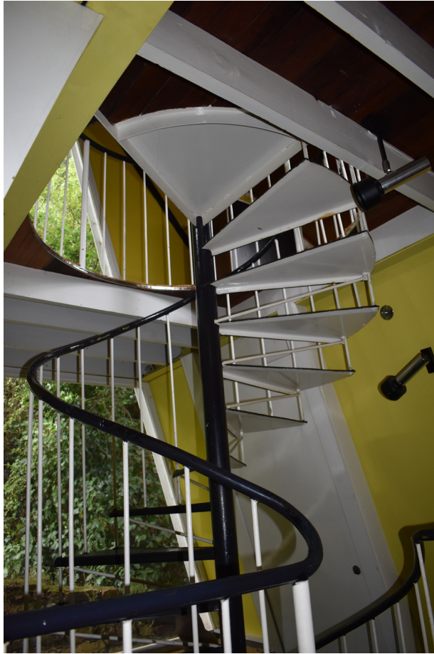
Figure 4. Spiral staircase. Note original front door in 'open' position against wall.
