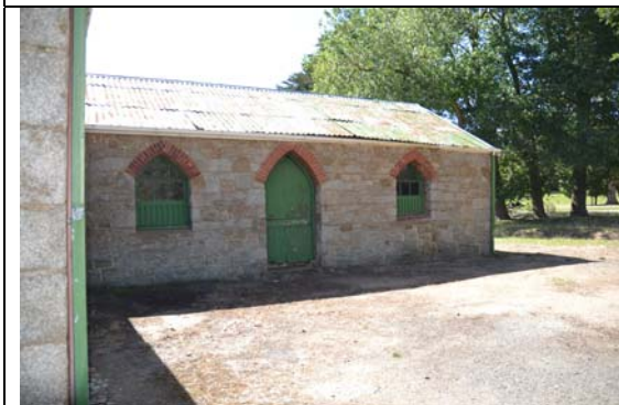
Photo 5 West wall of main gable.
