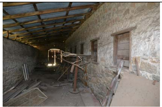
Photo 42 Store (Room 5) Looking south showing openings in west wall.
