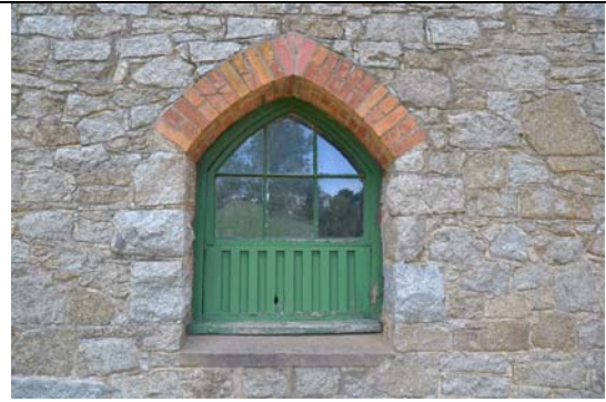
Photo 2 Detail of window, west gable end showing timber vent in lower section
