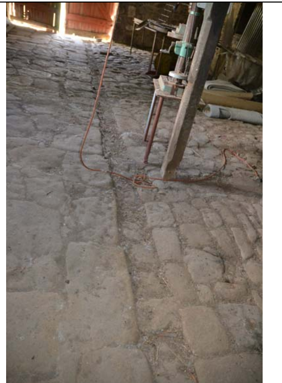
Photo 36 Stables (Room 3) showing detail of central drain in cobble floor.
