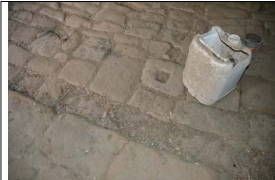
Photo 37 Stables (Room 3) Detail of squared stone at base of stall post.
