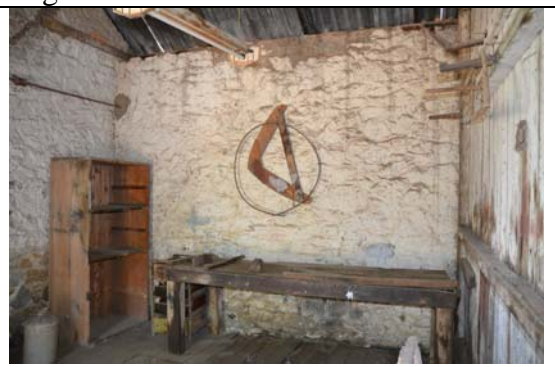
Photo 20 Interior of Tack Room (Room 1) looking north. Hanging pegs possibly for saddles and harness can be seen on the right.
