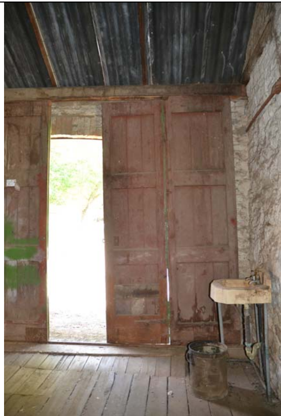
Photo 23 Interior of Tack Room (Room 1) looking south to doorway
