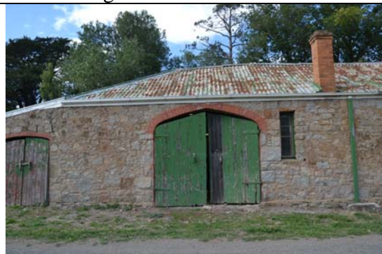
Photo 15 North wall showing doors to stables
