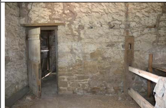
Photo 41 Loose Boxes (Room 4) Looking north to door to stables (Room 3)
