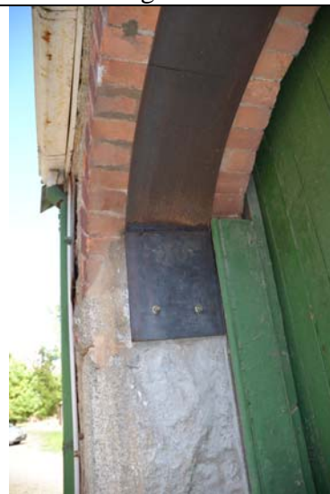
Photo 4 South face of west gable showing detail of door reveal showing curved stonework indicating earlier swing doors. Note introduced metal lintel.
