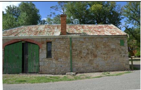
Photos 16 North wall , west end.
