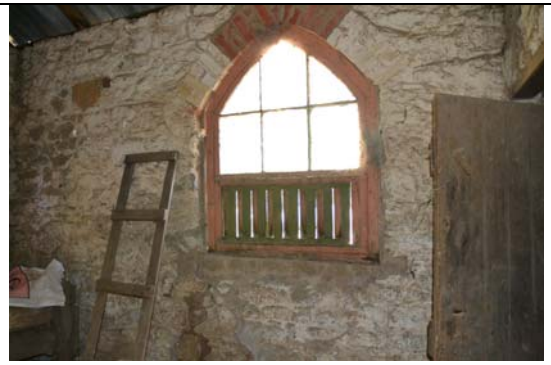
Photo 40 Loose Boxes (Room 4) Looking east showing window with timber vent below
