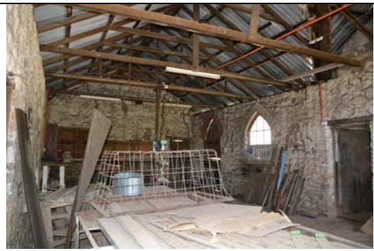
Photo 30 Stables (Room 3) looking south west showing external door and window and internal door to Grooms' Room (Room 2)
