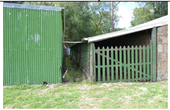
Photo 12 North wall, east end showing skillion extension over open area
