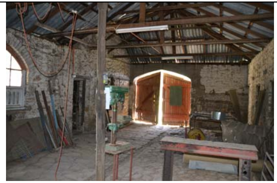
Photo 34 Stables (Room 3) looking north west to external double doors.
