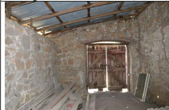
Photo 43 Store (Room 5) Looking south to external door.
