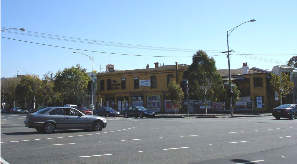
Figure 44 Nineteenth century development (including former Lemon Tree Hotel), at corner of Rathdowne and Grattan Streets, diagonally opposite the north-west corner of the REB site.
