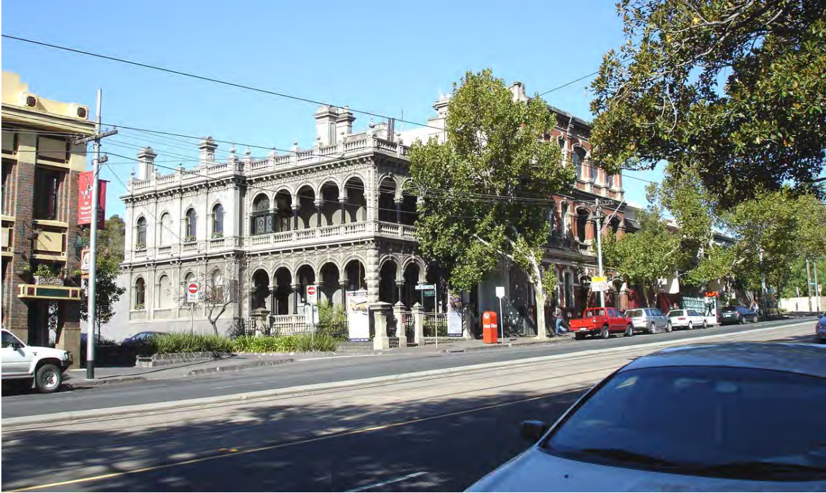
Figure 41 Nineteenth century development on Nicholson Street, opposite REB site.
