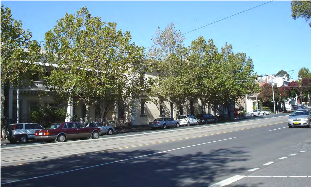
Figure 42 Nineteenth century development on Nicholson Street, opposite REB site.
