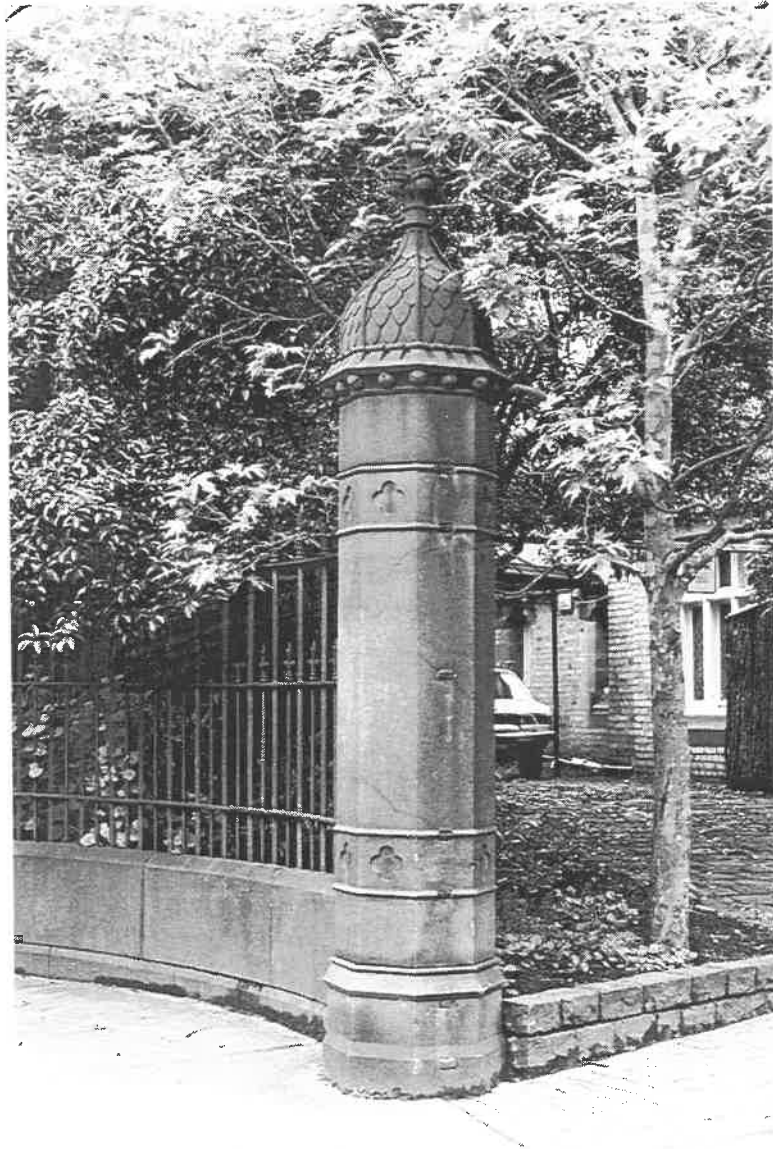
Photo 20. One of the surviving Pillars (on west side) (Note the iron fixing lugs, all that remain of the footpath gate) (Photograph taken October 1995)
