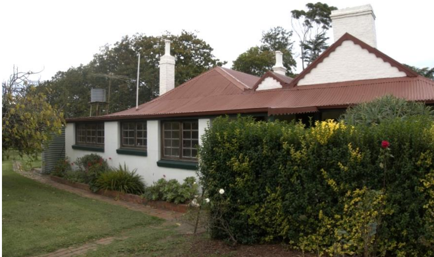
Figure 26. West (rear) elevation of the house, showing later extension of roof beyond line of the verandah
