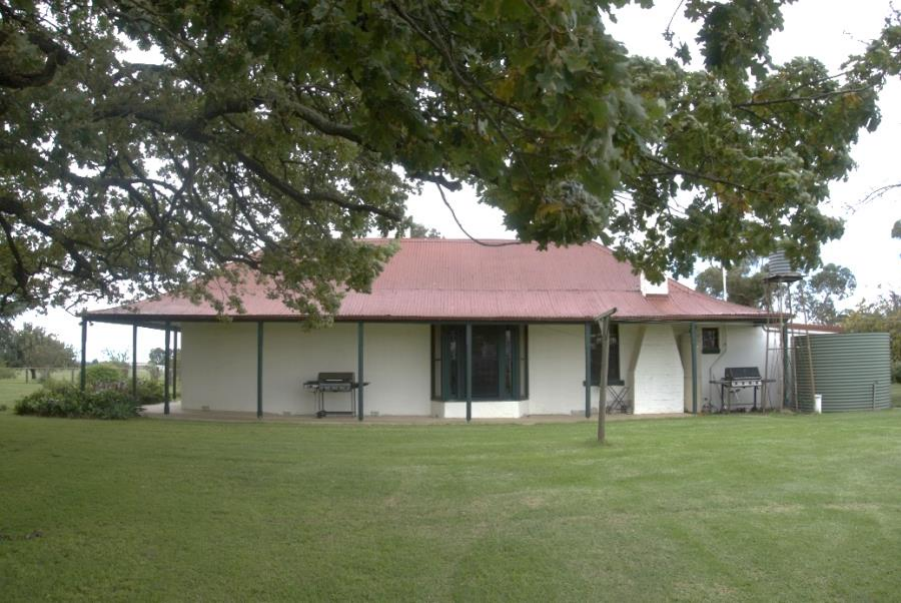
Figure 23. North elevation of the house
