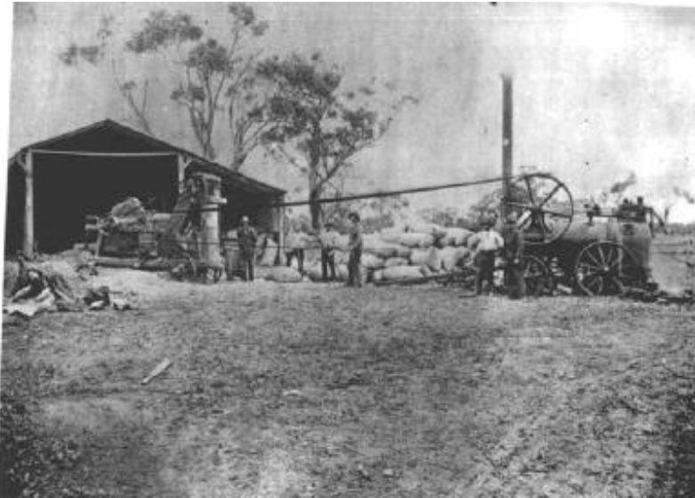
Figure 13. A Manks family chaff cutting machine, undated (Cranbourne Historical Society, included in City of Casey Thematic Environmental History, Context , 2004, p. 28)
