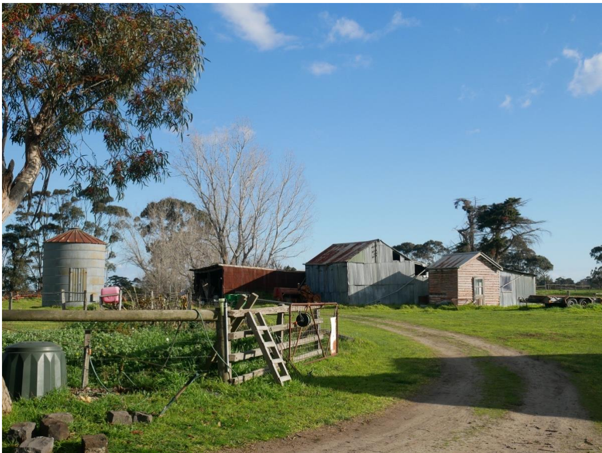
Figure 19. Collection of early outbuildings from the west (GJM, 5 August 2019)
