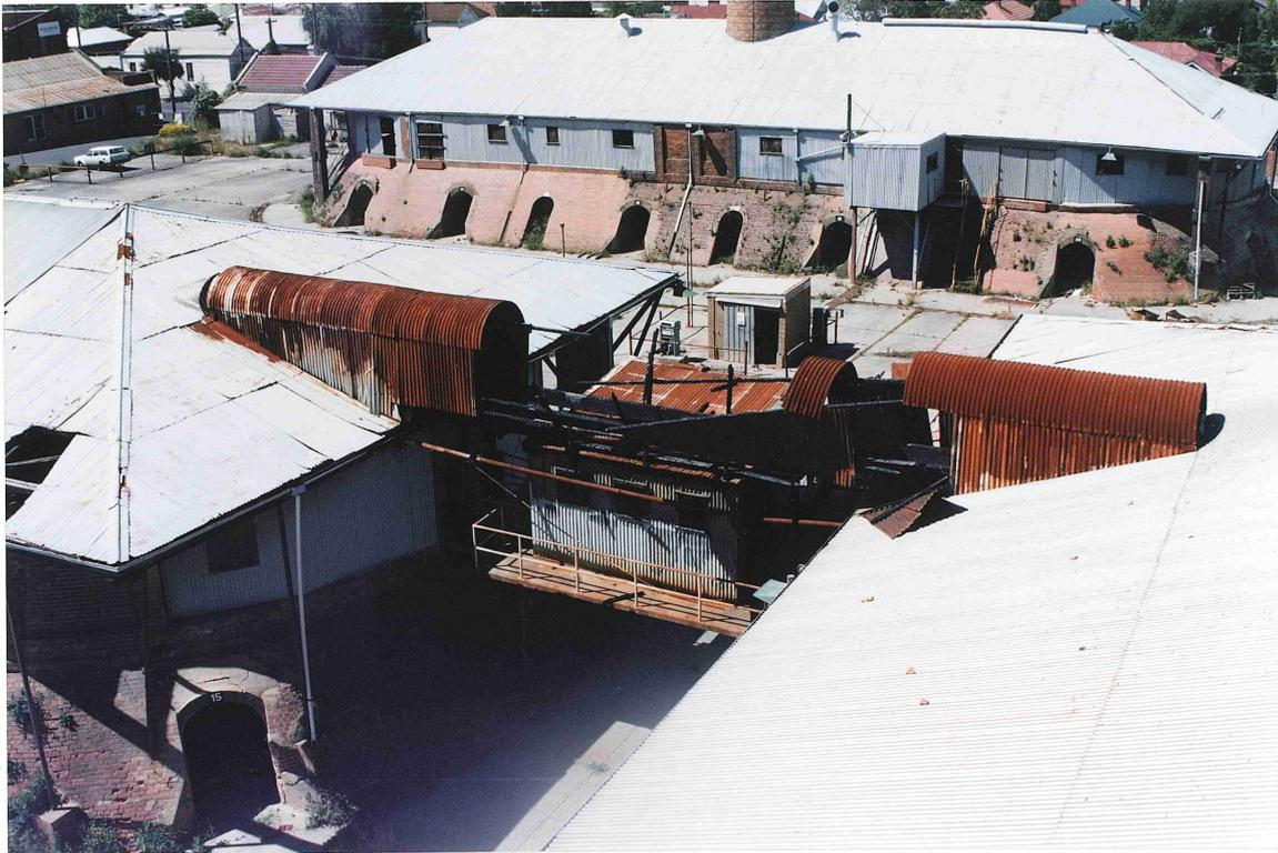
Figure 14. Building 4. Remnants of the crypto oil firing building which powered Kilns 1 and 2.
