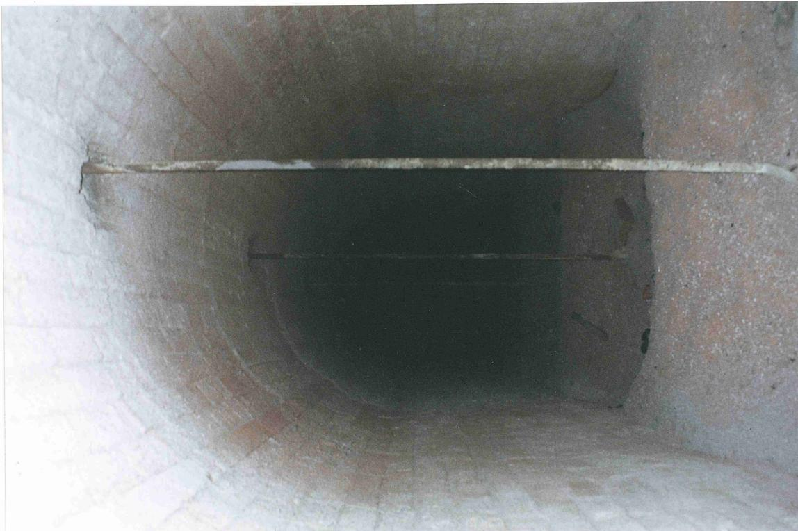
Figure 13. Hoffman Kiln 2. Photograph shows tunnel system and damper
