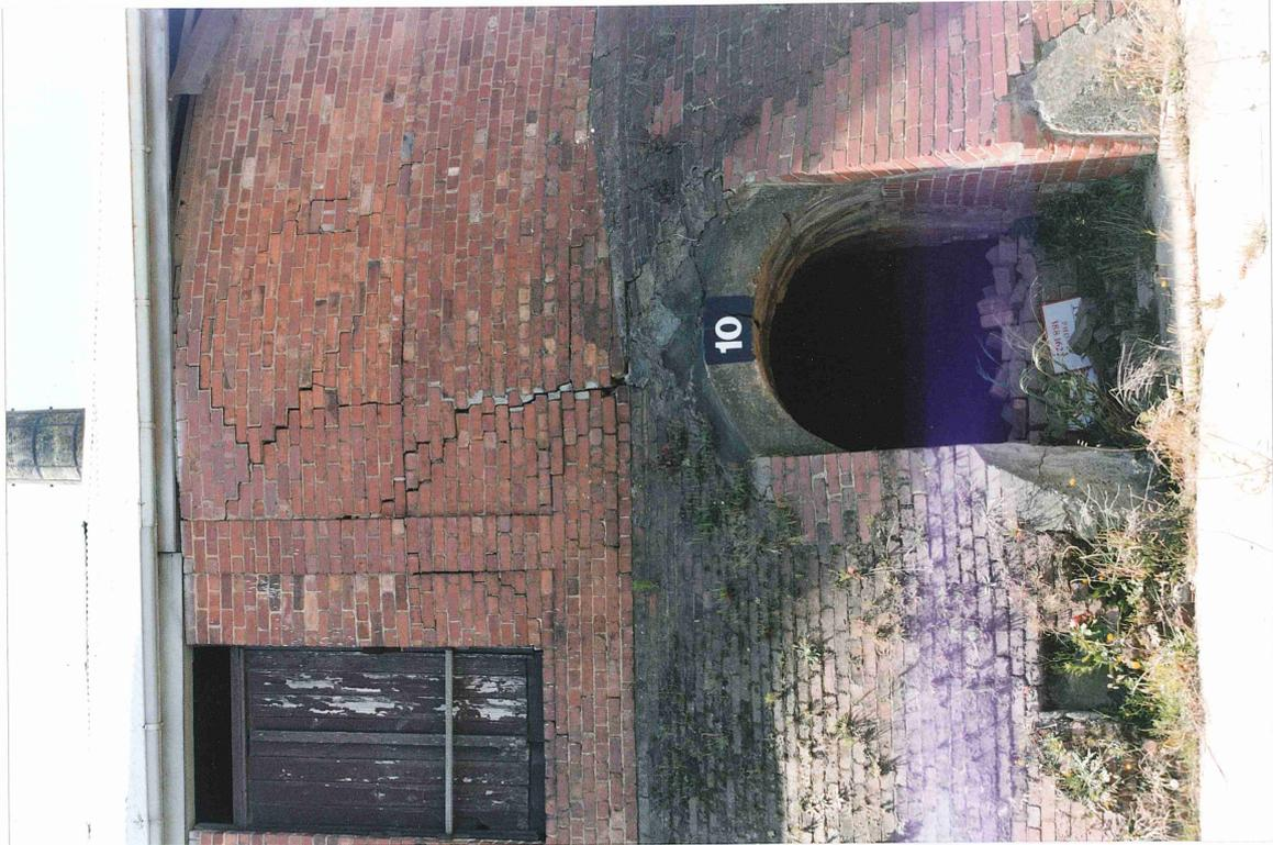
Figure 10. Hoffman Kiln 2. Photo shows modified wicket and cracking associated with brickwork panels to upper level of the kilns. Taken by Helen Lardner and Iain Stuart.
