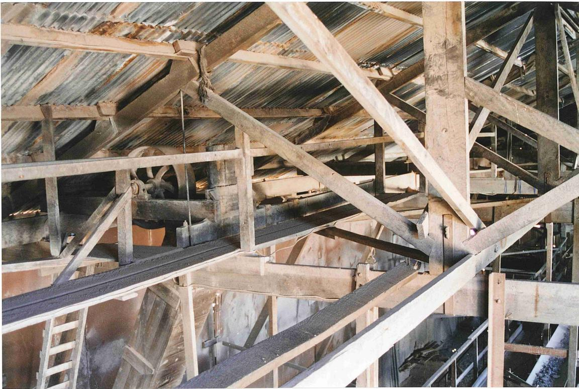
Figure 16. Building 5 - loft level. Photograph shows the equipment for moving material from Building 7 to Building 5 and the adhoc roof structure of the Brick Press Building.
