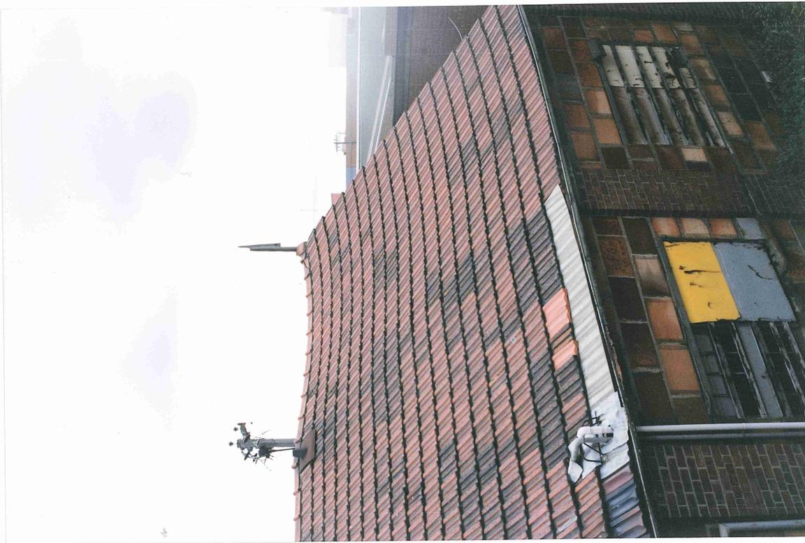
Figure 22. Building 17. Photograph shows the building's sagging roof structure and the hollow glazed blocks to the walls
