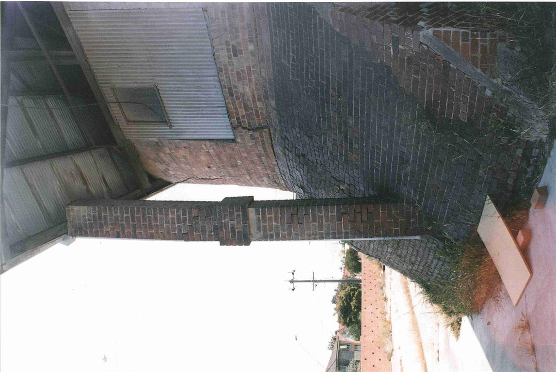
Figure 12. Hoffman Kiln 3. Photo showing structural failure to brick pier.
