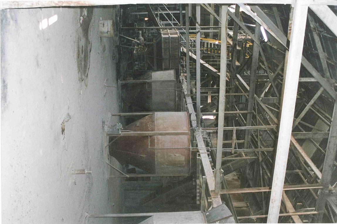
Figure 18. Building 5 - first floor level. Photograph shows timber building structure and hoppers.
