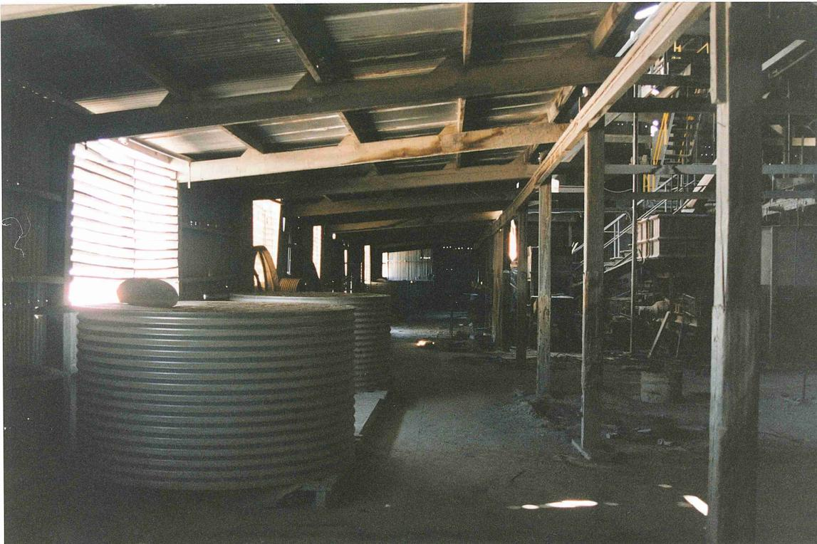
Figure 19. Building 5 - first floor eastern annexe. Photograph shows the separate roof structure and corrugated iron storage tanks.
