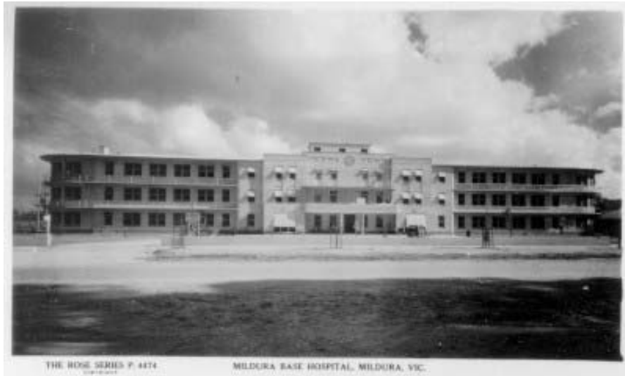
Mildura Base Hospital of 1934 by Irwin & Stevenson. This hospital is illustrative of the approach to health in which patients recuperate on sunlit balconies or in solaria, well lit rooms at the ends of the ward wings.
