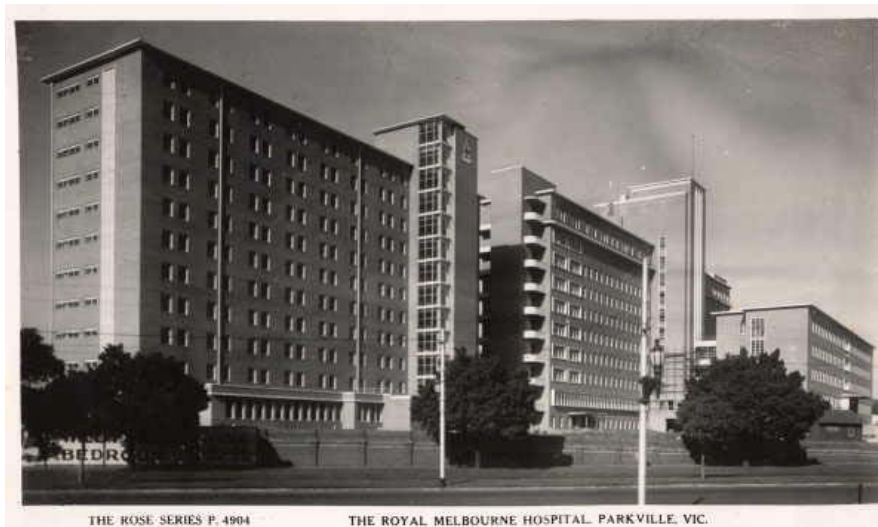
Royal Melbourne Hospital by Stephenson & Turner. The sunlit balconies have been replaced by sunhoods defining the architectural aesthetic of the building.
