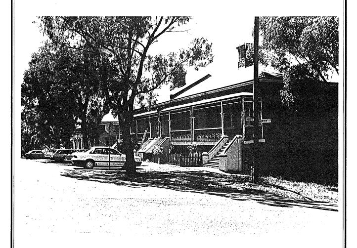
**3-19**Fernville Terrace, 35-41 Mackenzie Street, 1885; demonstrating the influence of the steep terrain on house design in this part of Bendigo where sub-basements become full height on the downhill side of a site.
