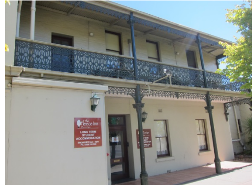
Fleece Inn, 143 Charleston Road, detail of front verandah
