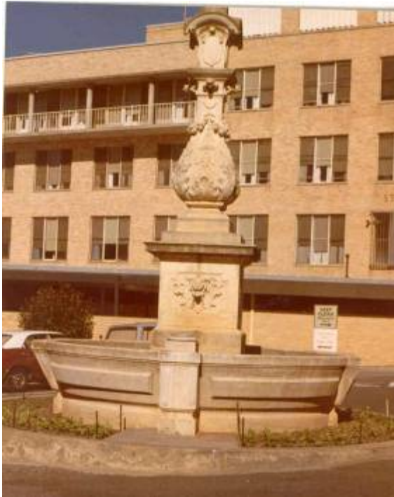
The fountain in front of the Central Block, before it was relocated, 1972. Source: Bendigo Health Records
