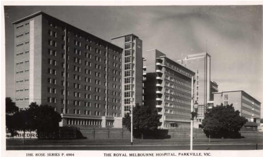
Figure 30 Royal Melbourne Hospital by Stephenson & Turner. The sunlit balconies have been replaced by sunhoods defining the architectural aesthetic of the building.
