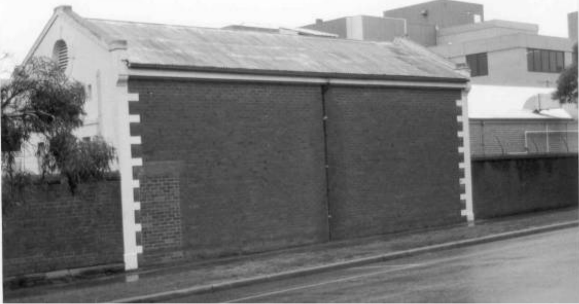
The Mortuary prior to restoration works, 1997. Note that the boundary walls abutted the building. Source: Bendigo Health Records
