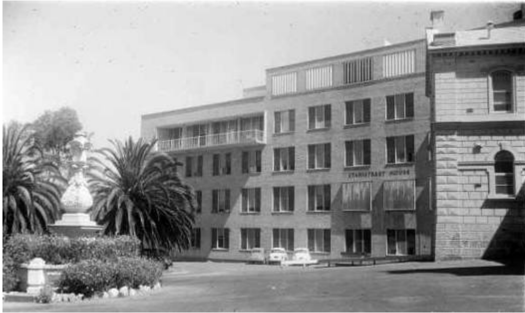
Undated photo taken prior to the construction of the Outpatients/Admissions building around the base of Stanistreet House in c.1964. Source: State Library Victoria
