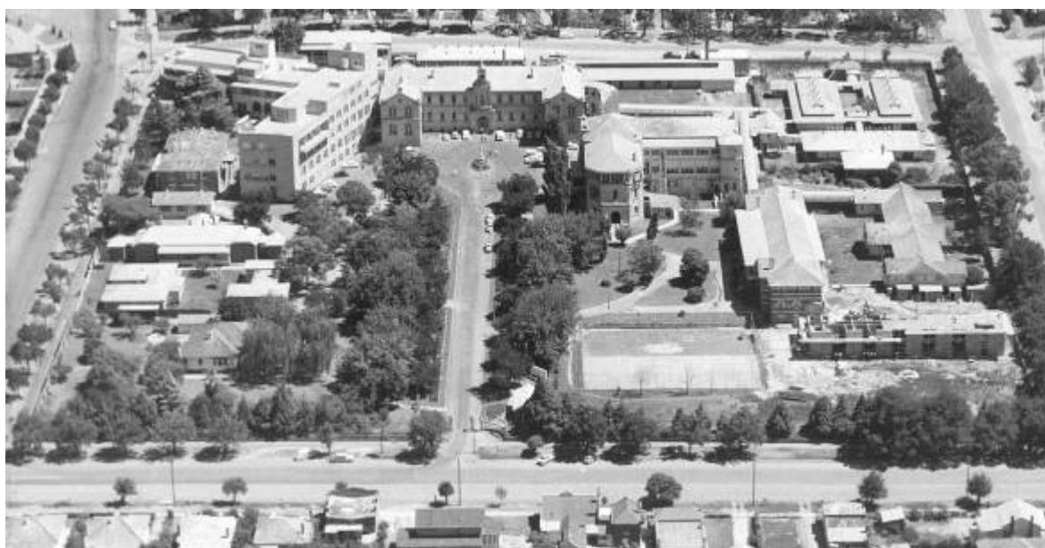
Trees lining the central driveway and boundaries in c.1963. Source: Bendigo Health Records
