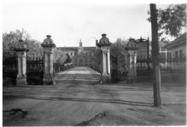
Figure 28 Bendigo Hospital, undated photograph.
