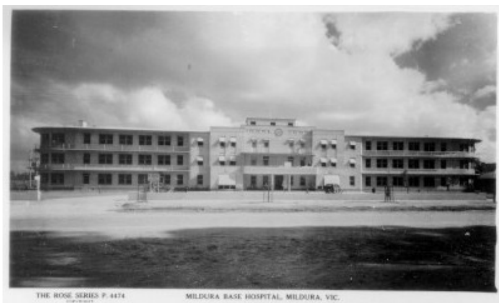
Figure 29 Mildura Base Hospital of 1934 by Irwin & Stevenson. This hospital is illustrative of the approach to health in which patients recuperate on sunlit balconies or in solaria, well-lit rooms at the ends of the ward wings.
