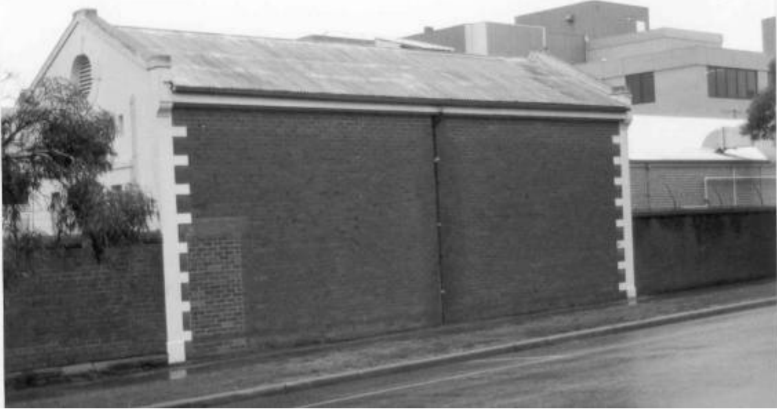
The Mortuary prior to restoration works, 1997. Note that the boundary walls abutted the building. Source: Bendigo Health Records
