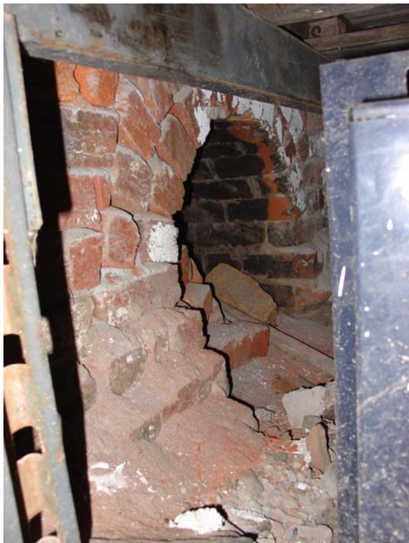
View of flue entrance on south side of chimney
