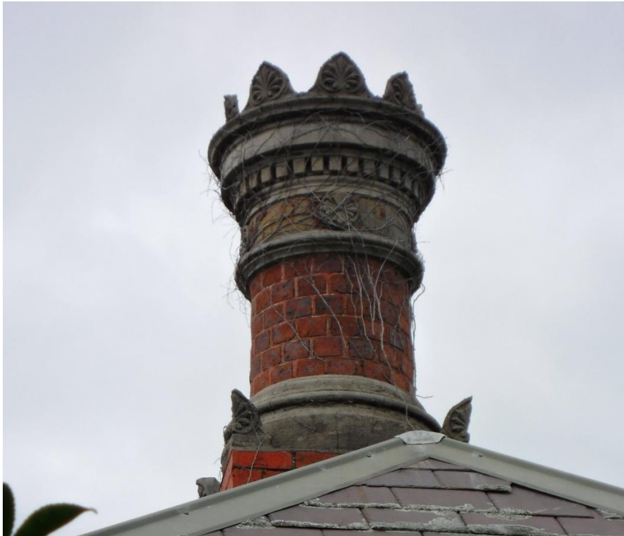
Figure 4. Front chimney. (Source: Context 2016)
