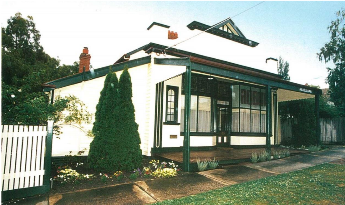
Figure 1. The front of the shop in 2002. Note the clear glazing to the shop windows and absence of a verandah frieze. (Source: Karen Gornalle & Associates, 2002)
