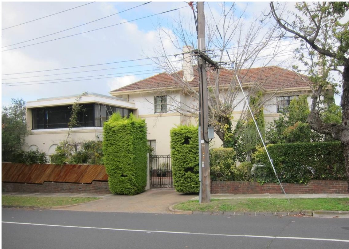
Figure 1. 486 Burke Road, seen from Pine Avenue. Source: Context Pty Ltd 2016.
