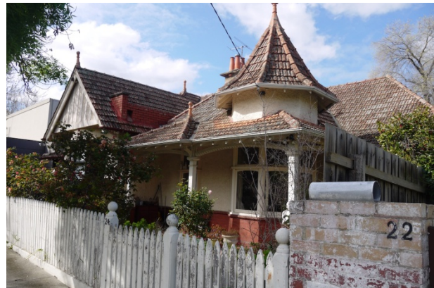
Figure 3. No 24 verandah and bay window detail (GJM Heritage/Purcell, June 2016)
