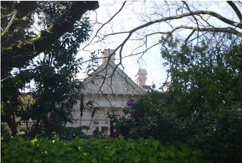
Figure 5. Gable and chimney detail (GJM Heritage/Purcell, June 2016)
