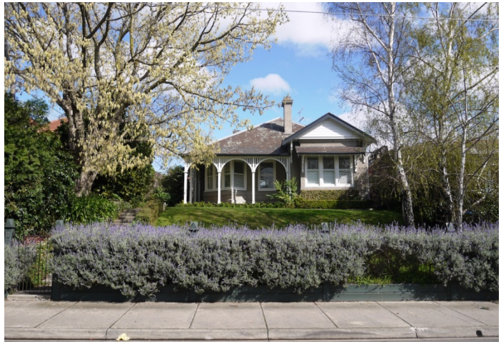
Figure 3. Facade of the house and deep setback (GJM Heritage/Purcell, June 2016)
