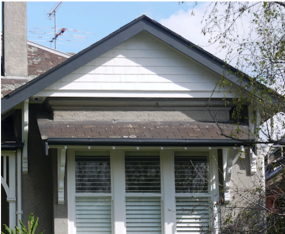
Figure 2. Gable end detail (GJM Heritage/Purcell, June 2016)
