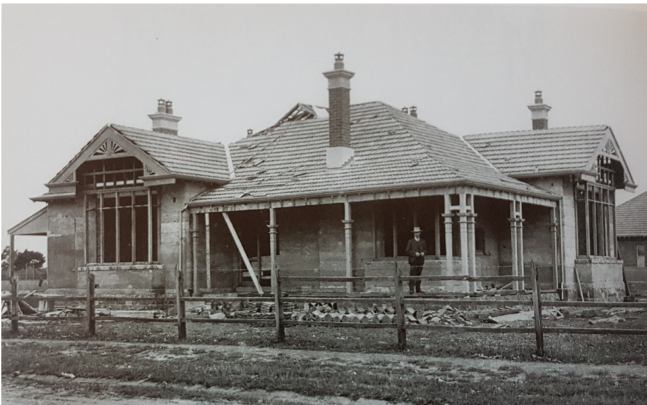
Figure 2. A villa under construction in Mont Albert Road, Canterbury, constructed using Crawford's patented hollow reinforced concrete wall system; not known if remains (Lewis 1988:26).
