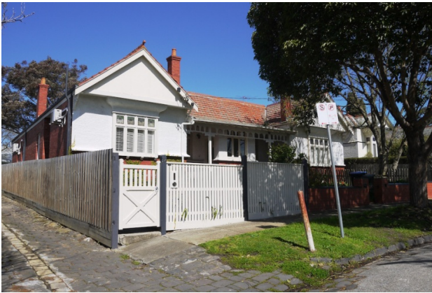
Figure 3. Entrance to No. 24 visible along the western elevation (GJM Heritage/Purcell, June 2016)
