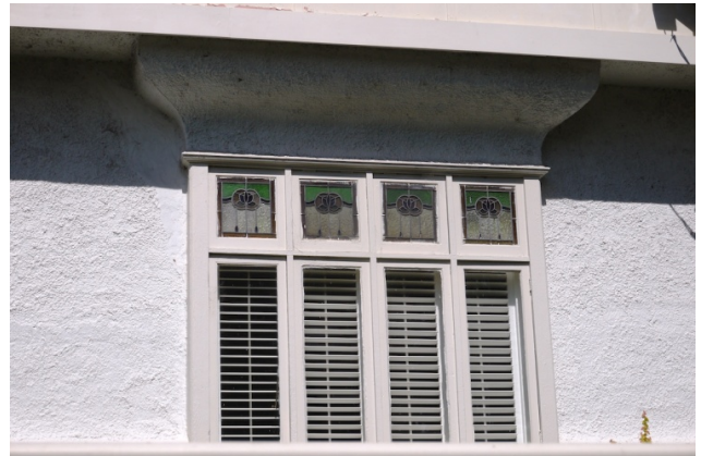
Figure 4. Window detail (GJM Heritage/Purcell, June 2016)
