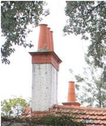
Figure 4. Chimney detail (GJM Heritage/Purcell, June 2016)
