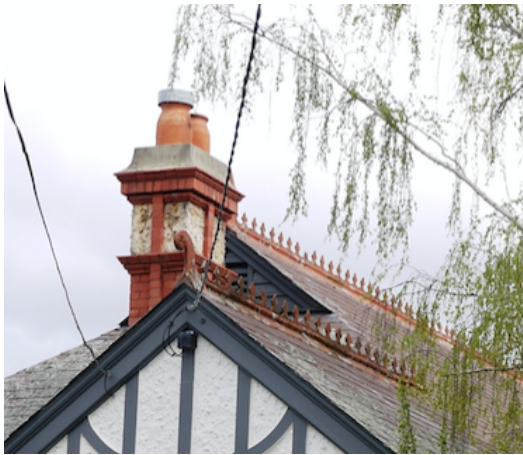
Figure 4. Roof and chimney detail (GJM Heritage/Purcell, June 2016)
