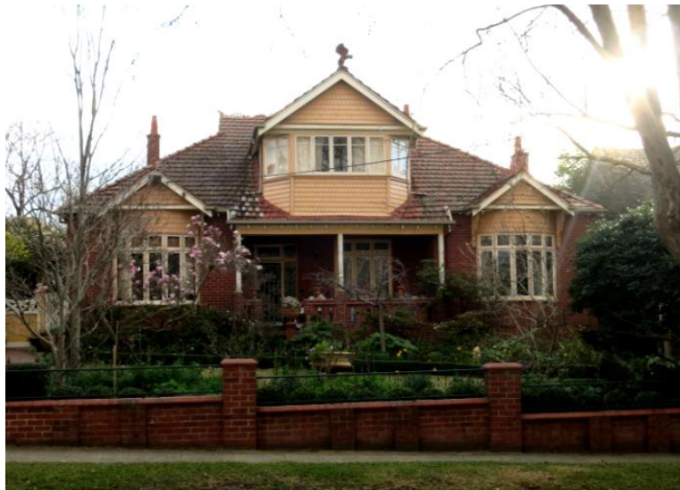
Figure 1. 123 Finch Street (GJM Heritage/Purcell, June 2016)
