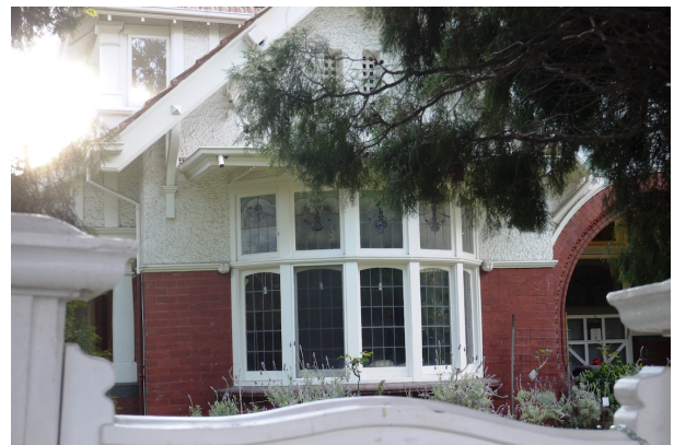
Figure 5. Bow window detail with vented gable above (GJM Heritage/Purcell, June 2016)
