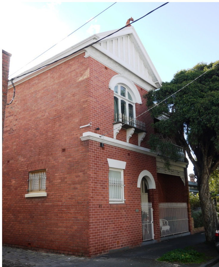
Figure 1. 41 Perth Street, Prahran (GJM Heritage/Purcell, June 2016)
