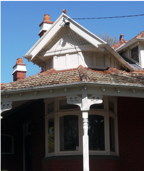
Figure 2. Gablet, bay window and verandah detail (GJM Heritage/ Purcell, June 2016)
