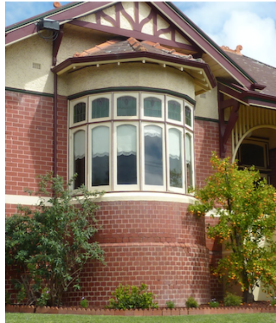
Figure 4. Bay window detail (GJM Heritage/Purcell, June 2016)
