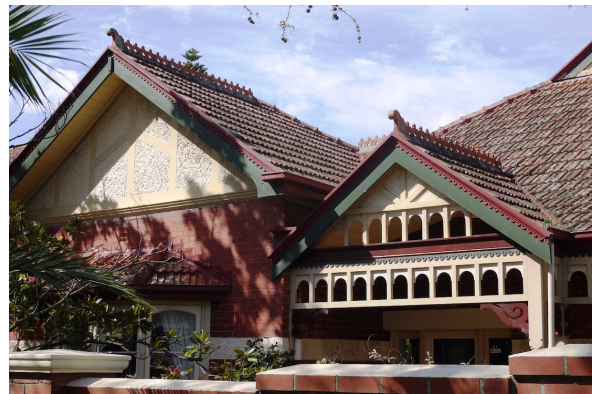
Figure 5. Gable end and verandah detail (GJM Heritage/Purcell, June 2016)
