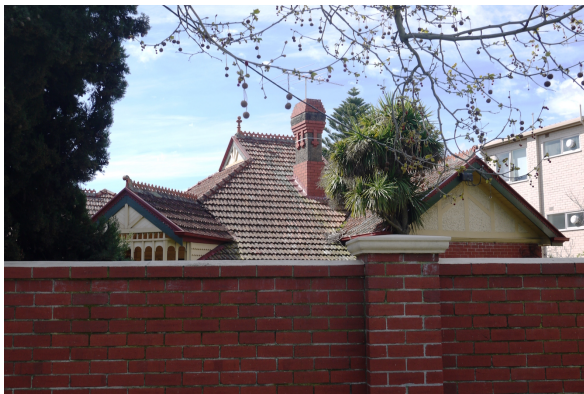
Figure 4. Roof and chimney detail (GJM Heritage/Purcell, June 2016)
