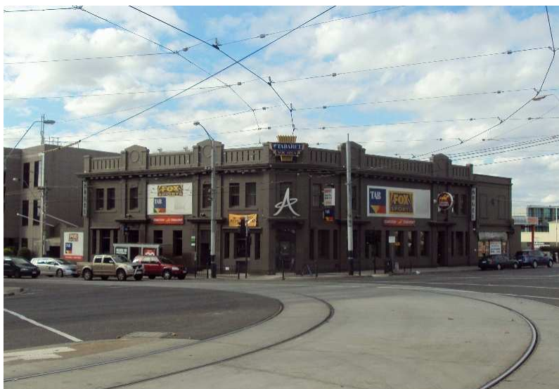
Former Railway Hotel
