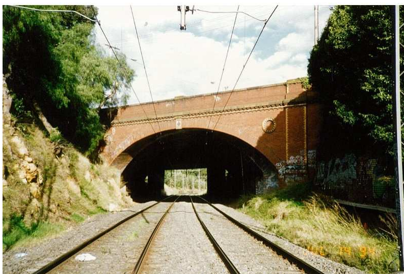
Dandenong Road Bridge. Source; National Trust of Australia (Victoria)
