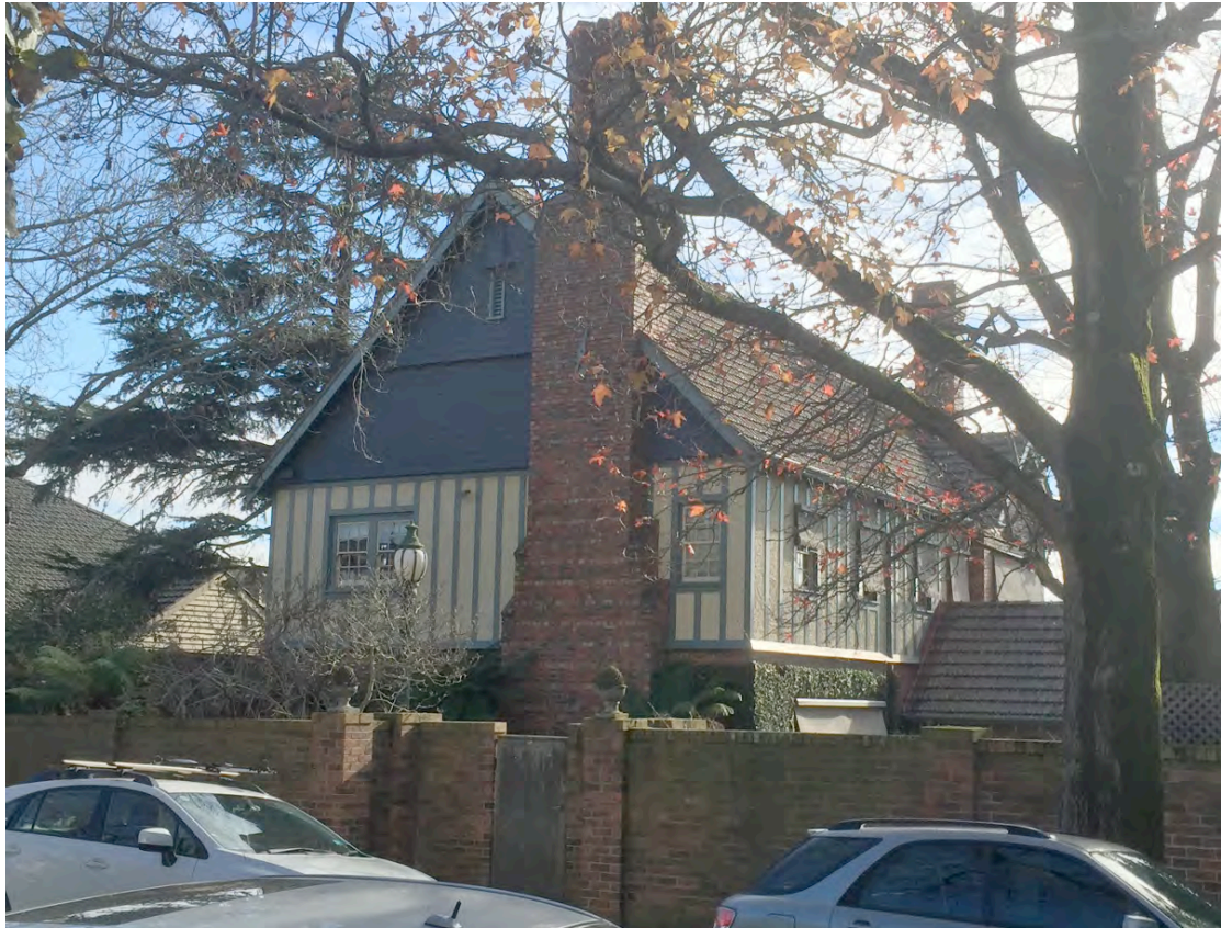
Figure 1 1 Chesterfield Avenue, Malvern.
