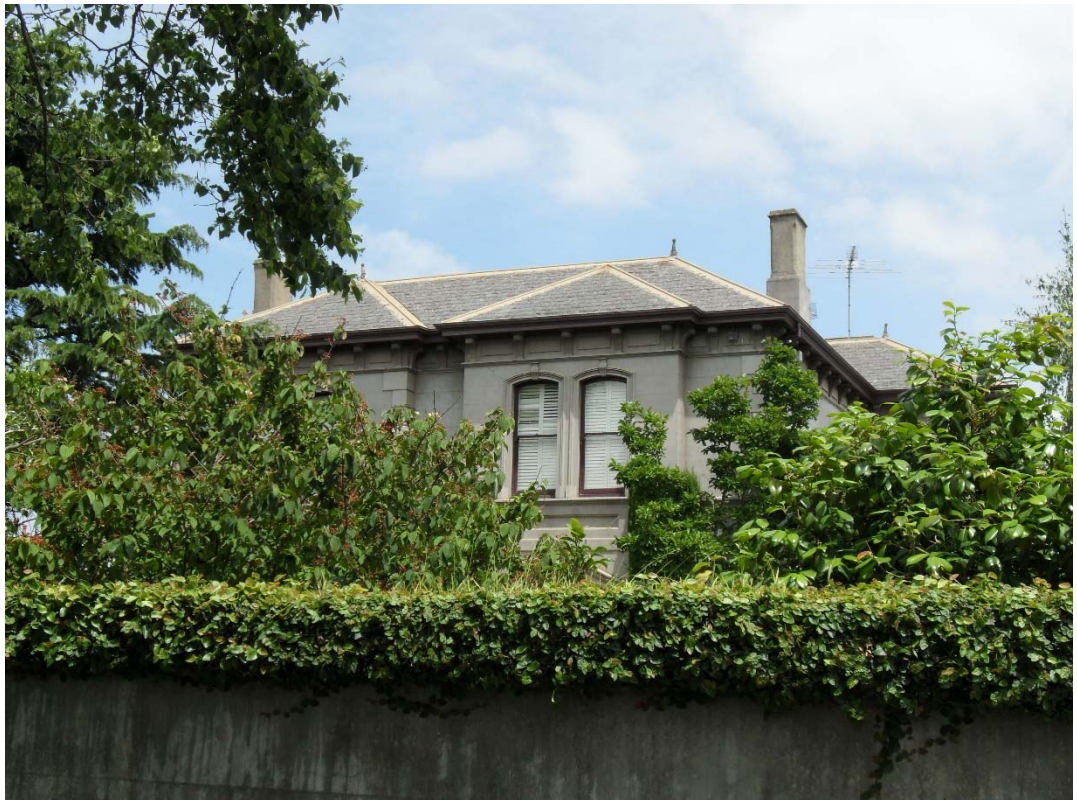
Figure 3. Front façade of ‘Nauroy’, showing the two breakfronts, hipped roof, and truncated chimneys. (source: Context, 2016)
