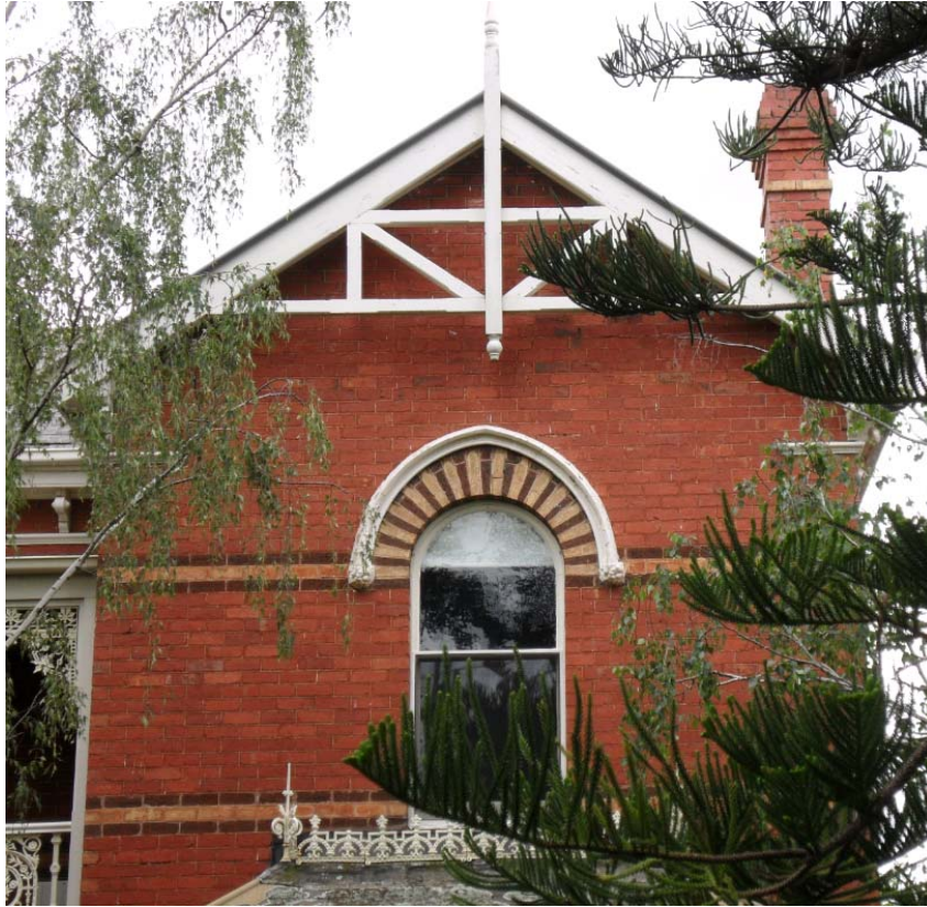
Figure 6. Detail of the front projecting gable, with the timber trusswork, Venetian Gothic window. The cast-iron crest to the bay window below is not an original feature. (source: Context 2016)
