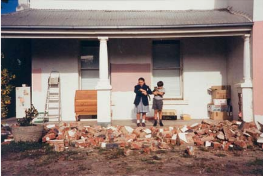
Figure 4. Front verandah of 50 Elizabeth Street in 1992, showing the interwar verandah supports and the original ogee-profile roof. (source: Stonnington History Centre, Reg. MP14527)
