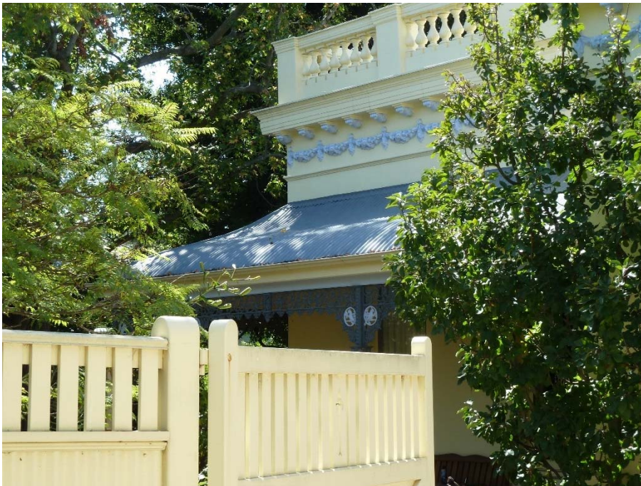
Figure 6. Detail of balustraded parapet and elaborate cornice at 'Gracedale' at 50 Elizabeth Street (source: Context 2016).
