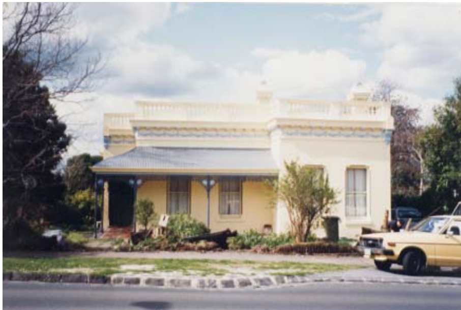
Figure 5. House at 50 Elizabeth St, Malvern, taken in 1992 (Stonnington Library and Information Service).
